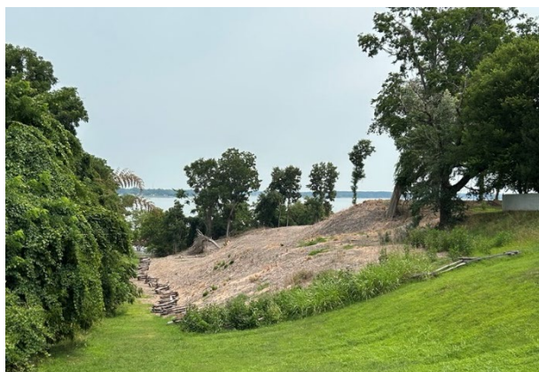
Yorktown's Great Valley Road before (top) and after (bottom) bamboo areas were treated and removed.
