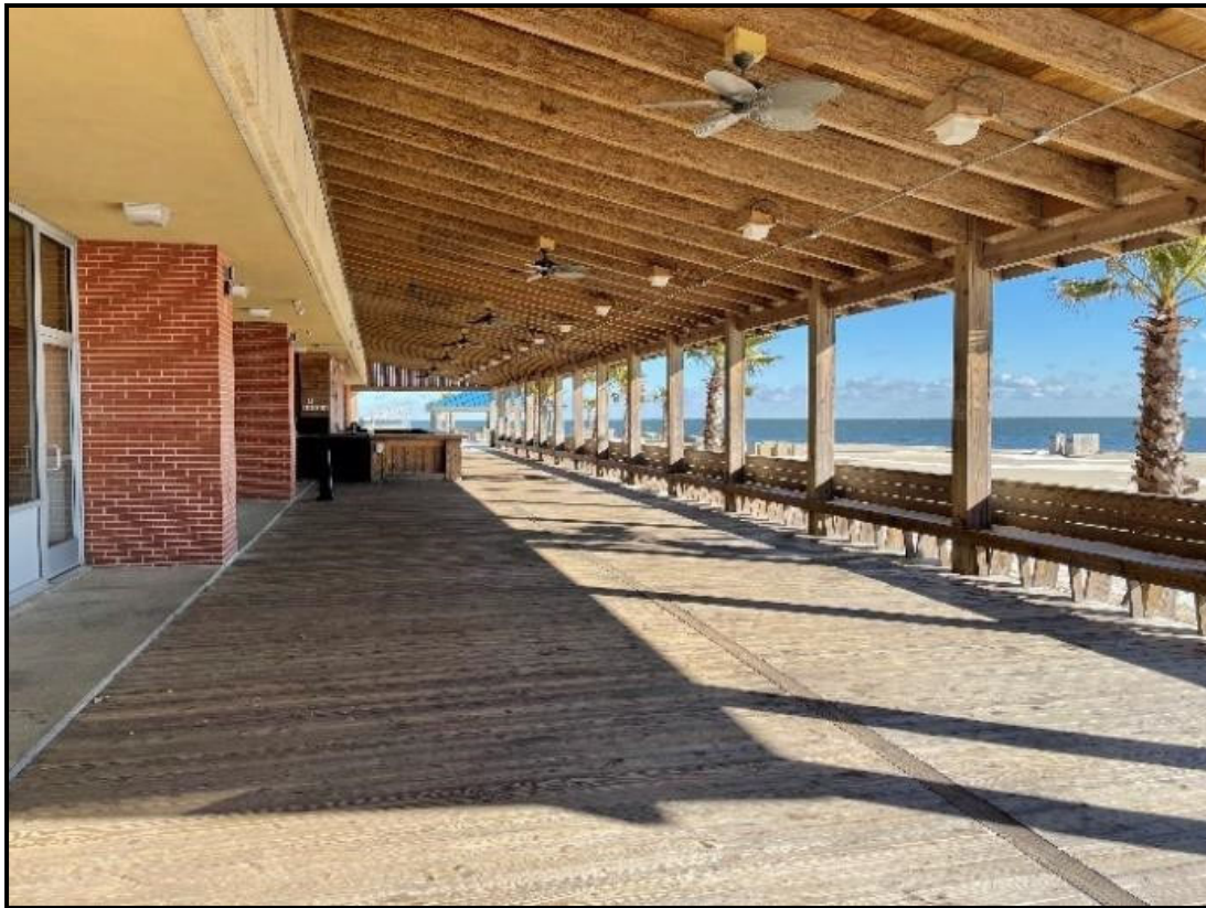
(Back Deck View at Ft Monroe Multi-Use Facility)
