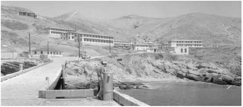
Air Force base at Johnsons Lee seen from the pier, August 1965.
