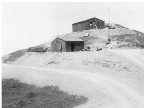
Army radar buildings, 1944.
