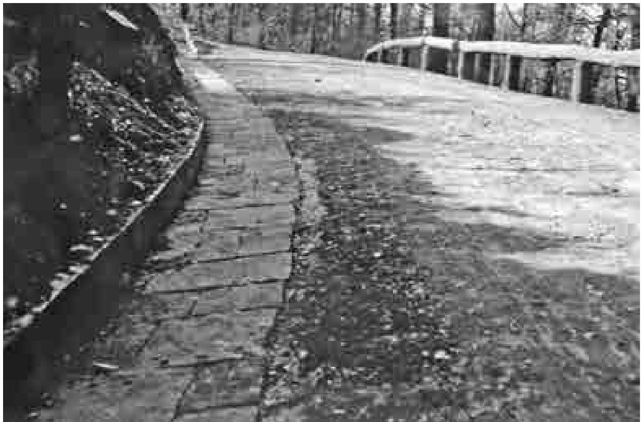
Figure 2.34: "Old Cravens Road - Fine Grading and Rip Rap - After," 1937. (CHCH Archives)
