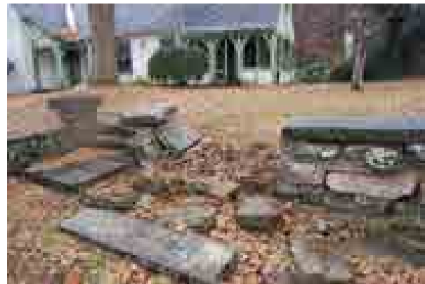
Figure 3.28: Failure of Williams House Fieldstone Retaining Wall (Lower). (The Jaeger Company, January 2011)
