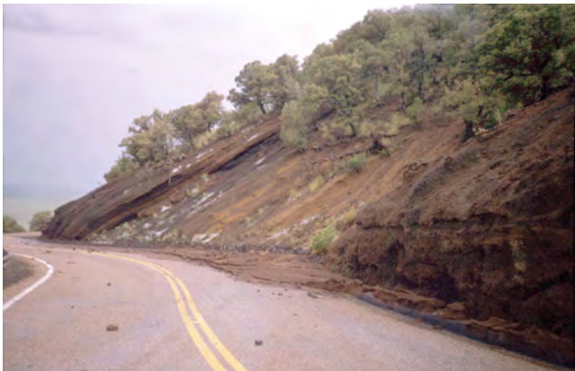
Figure 33. Photograph of slope movements along Volcano Road. Slope movements include fall, topple, slide, spread, and flow of material under the influence of gravity. Rockfall, slope failure, and small debris flows are common along Volcano Road. Slope-movement events occur on time scales ranging from seconds to years, and may be triggered by storms and higher-than-average precipitation. National Park Service photograph (date unknown).
