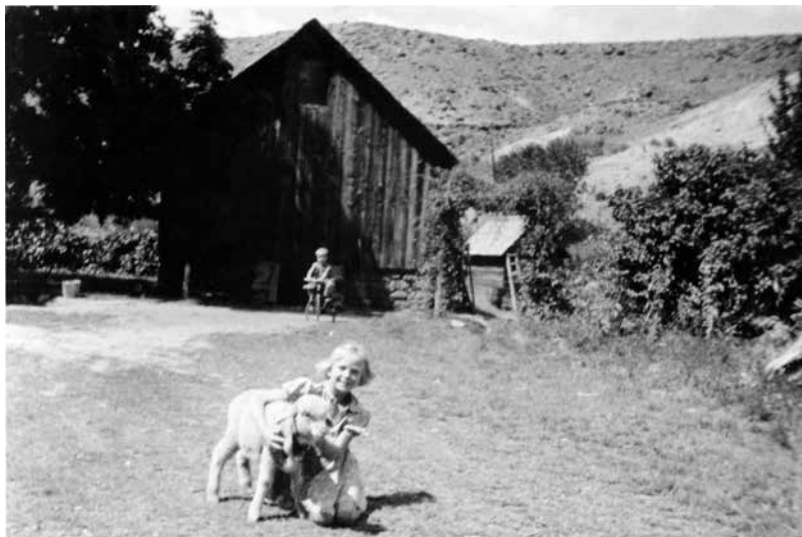
Twila Gifford plays with a lamb in front of her family's home in the late 1930s. Over the years, the house was remodeled into the building seen today.
