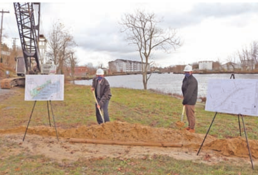
Ground was broken on phase one of the revitalization of the old J.B. Robinson Oyster House site along the Seaford River Walk. (Chesapeake Conservancy)
