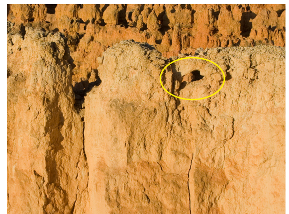
An ice window (circled) has formed along a joint in a fin near Sunset Point; to the left is a collapsed window along another joint - the beginnings of a new hoodoo.
