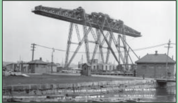
Floating Derrick No. 21 (YD-21)
