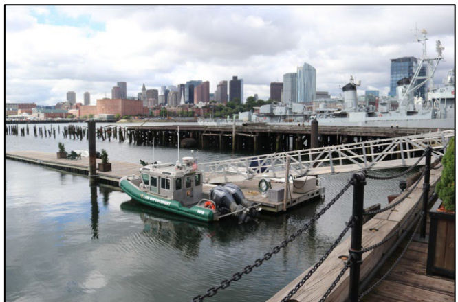
Pier and dock
