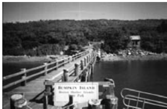
Pier for Water Shuttle
