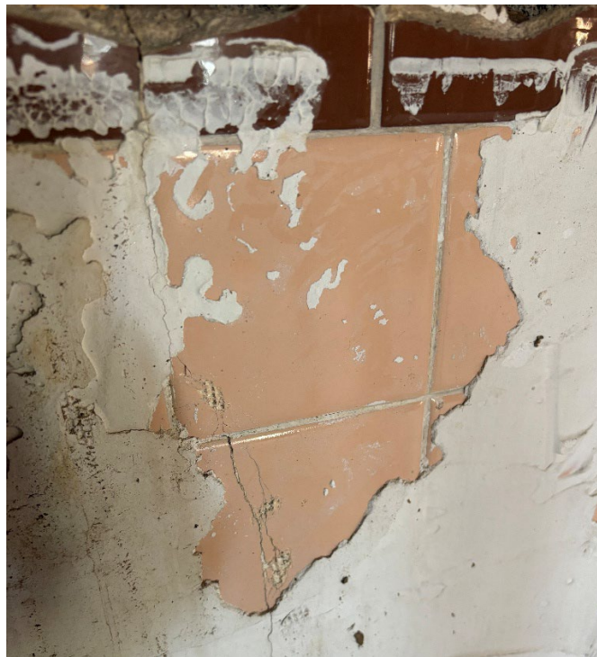
Figure 12 Existing wall tile, guest bathroom, A.G. Gaston Motel, August 21, 2024, History Associates.
