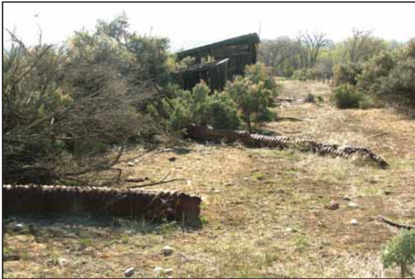
Culvert and Building Remnants
