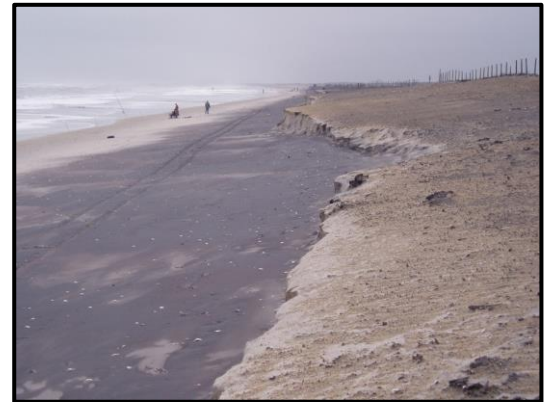
Beach erosion caused by high waters during a storm in 2009 [NPS]
