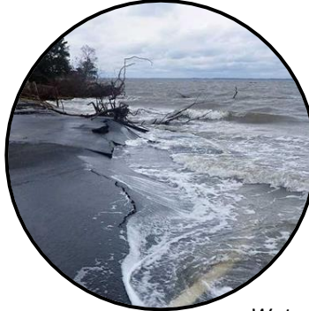
High storm surge during Hurricane Sandy damaged the Bayside Parking Area [NPS]
