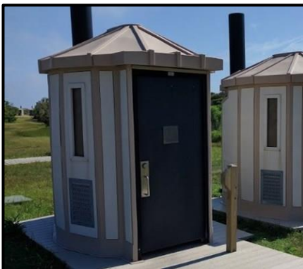
Moveable restrooms near the park's beach [NPS]
