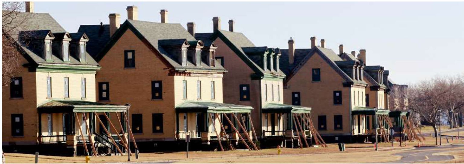
Buildings in Gateway National Recreation Area's Fort Hancock Historic Landmark District were devastated by Hurricane Sandy in 2012.
