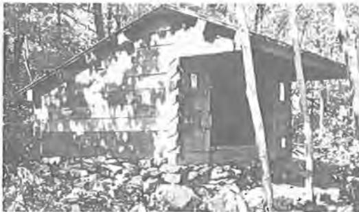
A solid, presawn and prefabricated construction was used in the Smith Shelter in Pennsylvania.
