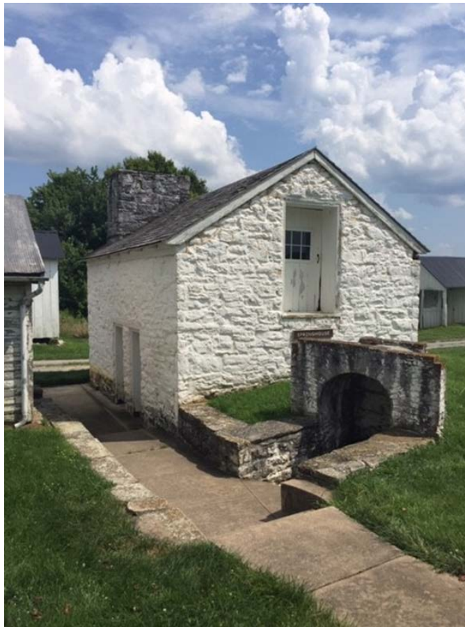
Mumma smokehouse with door on upper level to former slave quarters. (NPS)
