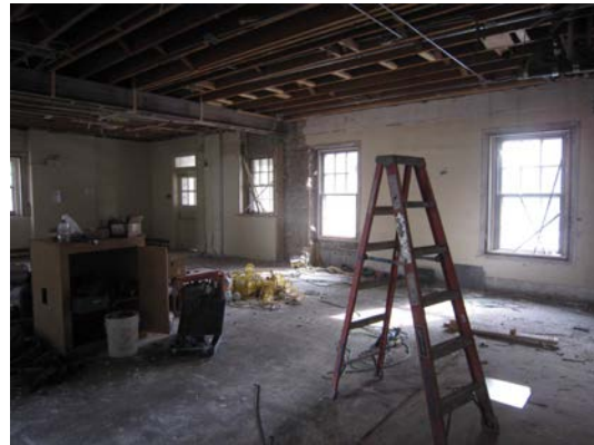
Interior view of rehabilitation for seismic and associated building work
