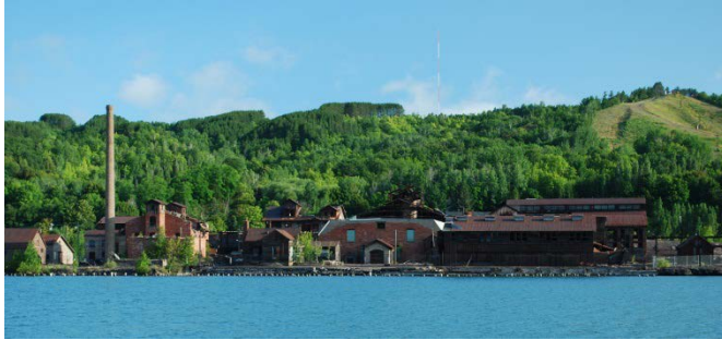
Ruins of the Quincy Smelter are located on Portage Lake across from the Houghton waterfront, Keweenaw NHP.
