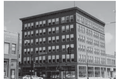
Marsh Place Building
