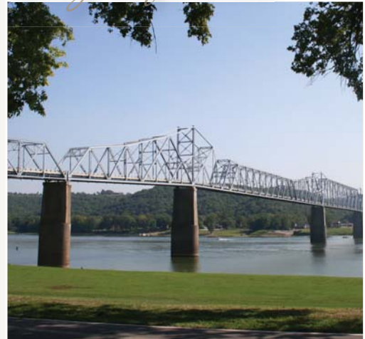
Milton Madison Bridge over the Ohio River between Kentucky and Indiana (photo courtesy Wilbur Smith Associates/Michael Baker Engineers)
