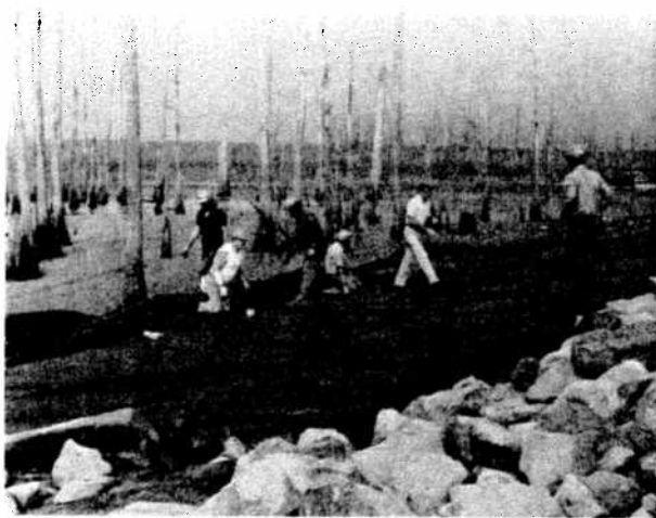
Placing filter cloth on Hurricane Mound in preparation for placing riprap, Sardis Lake, MS.
