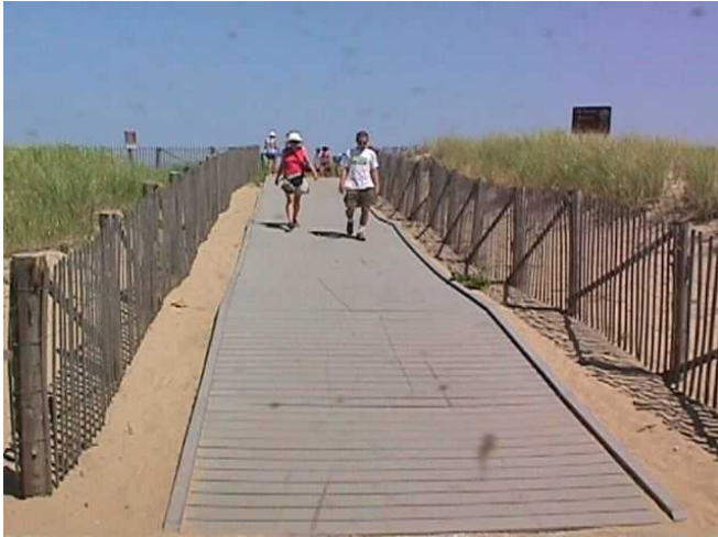
A recycled plastic boardwalk and installation of recycled paper countertops at Race Point Ranger Station
