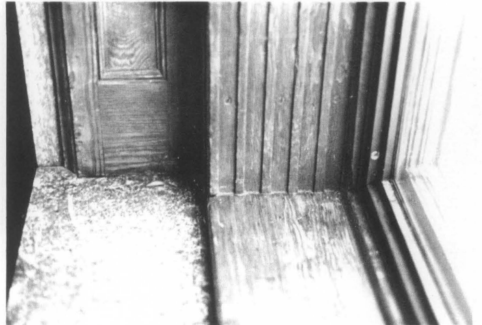
Figure 8. The decorative jamb panel on the left and the interior shutter tracks were unaffected by the installation of the interior storm window shown on the right. Photo: Charles E. Fisher
