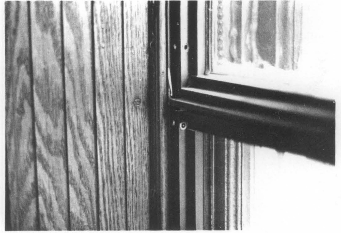
Figure 6. The windows were too large for only a single storm panel, necessitating the use of a structural subframe at the mid-section of the window. Both the upper and lower storm panels are operable and come together opposite the historic meeting rail. This element of the storm window is sufficiently thin that is not readily discernible from the outside. Photo: Charles E. Fisher
