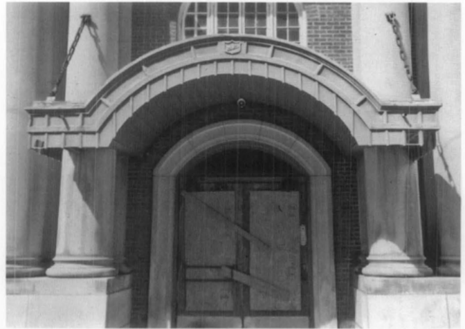
Figure 1. The Aldridge Hotel's south main entrance canopy as it existed at the start of the building's rehabilitation.
