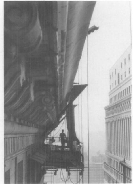
Figure 8. Access to the cornice was provided by cantilevered aerial scaffolds at the southeast and southwest corners of the cornice. All other locations were accessed by hanging two swing stages, side by side. The inner swing was hung off of a V-shaped bracket (shown) while the outer swing was hung from a steel deadman which projected horizontally across the cornice roof. Both the V-shaped bracket and the deadman were designed to transfer the weight of the swings vertically down through the center of the cornice. No load was placed on the outer edge of the cornice. Photos by Jeffrey S. Levine.
