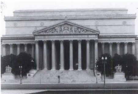
1. Completed in 1935, the National Archives is the repository for official Federal documents. Photo: Hugh Talman.
