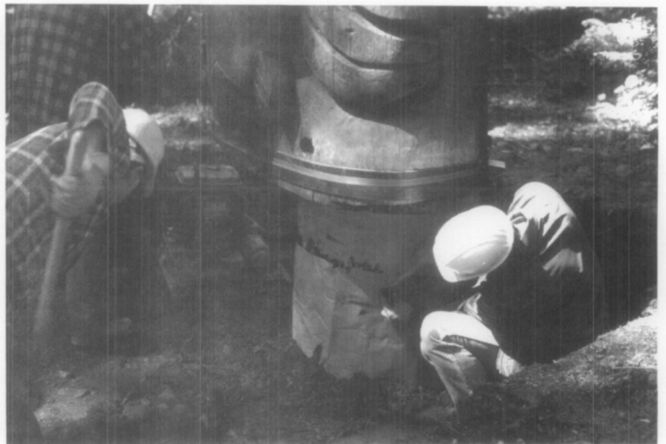
Figure 9. After securing the support post in the ground, a wood preservative in a "bandage" form was attached to the support post before dirt was filled to grade level.
