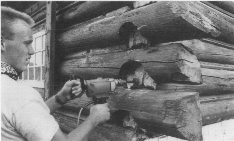
Figure 3. A plumber's bit was used to recess the crown back to the center line to create a flat surface for attaching the replacement crowns. Photo: Harrison Goodall.
