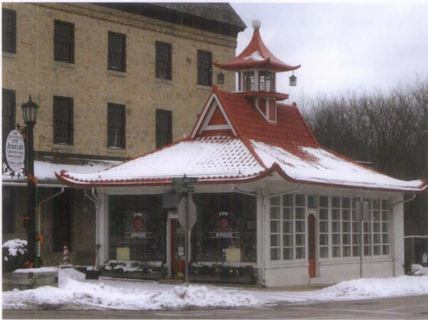
Figure 9. The dominant feature of this former gas station (1929) in Cedarburg, WI, is its pagoda-style metal tile roof (complete with upturned eaves and Japanese lanterns suspended from the cupola). The building currently functions as a jewelry store. Photo: Kenneth M. Itle, Wiss, Janney, Elstner Associates, Inc.
