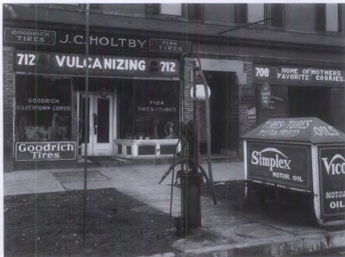
Figure 2. Although hardly an ideal sales system, pumps and underground tanks along the curb were an improvement over the earliest filling stations where gasoline was poured from hand containers. Photo: Utah State Historical Society, used by permission, all rights reserved.
