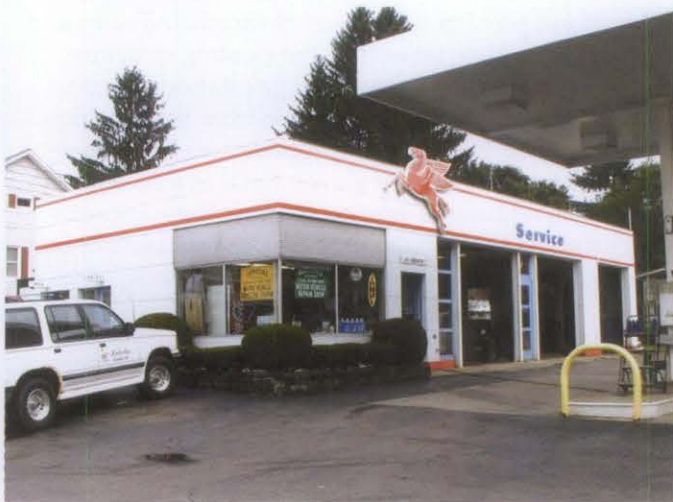
Figure 13. Essentially unchanged since its construction in 1950, this service station in Canisteo, NY, is currently owned and operated by the son of the original owner. Photo: Debra Jane Seltzer.
