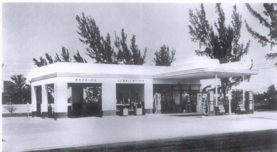
Figure 6. Box-type stations often incorporated Art Moderne forms such as this design's rounded corners, stripes, and large sales windows. Photo: American Petroleum Institute Photograph and Film Collection, Archives Center, National Museum of American History, Smithsonian Institution.
