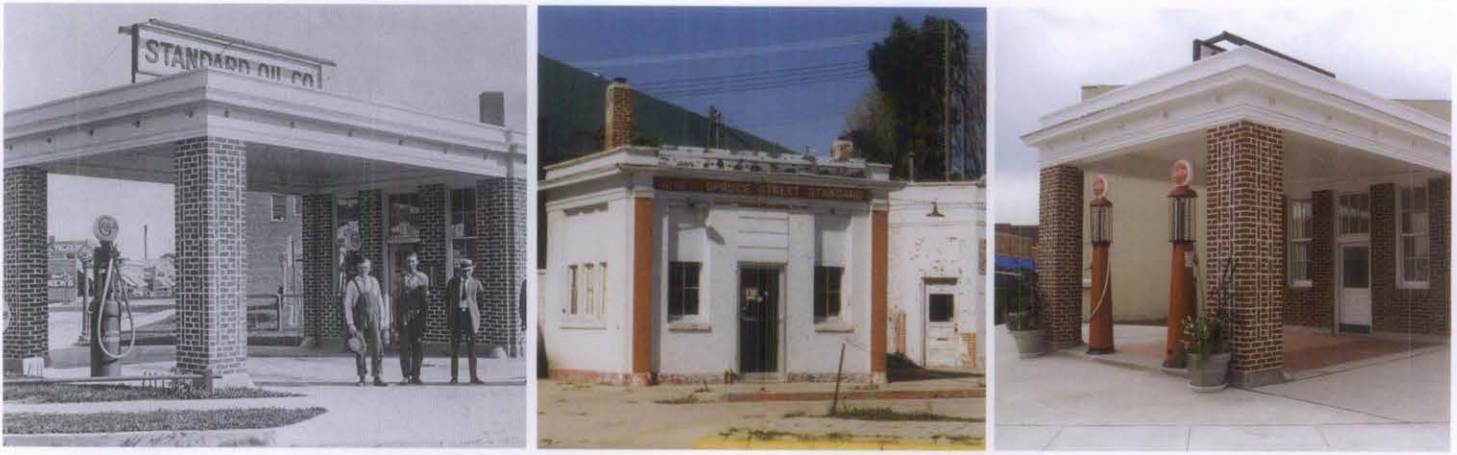
Figures 18. The canopy of the 1920s Spruce Street Station in Ogallala, NE, was an important feature that contributed to the building's character (left). When recently purchased for rehabilitation the canopy had long since disappeared (center). Using photographic and physical evidence, the canopy was reconstructed to match the building's original appearance (right). The station currently functions as a Main Street program office, a visitor center (on Nebraska's Western Trails Historic and Scenic Byway as well as Lincoln Highway Scenic Byway), meeting room, and public restroom facility. Photo: Ogallala Main Street.
