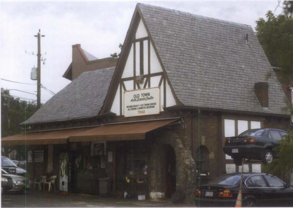
Figure 4. Designs based on popular domestic forms helped stations blend in with residential neighborhoods while imparting a sense of stability and permanence. This Tudor Revival station was converted for use as a repair shop with virtually no change to the structure or site.
