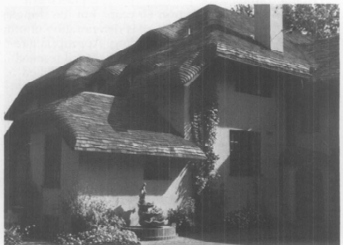
4. With the popularity of the revival of historic styles in the late 19th and early 20th centuries, a new technique was developed to imitate English thatch roofs. For the Tudor Revival cottages, steaming and curving of sawn shingles provided an undulating pattern to this picturesque roof shape. Photo: Courtesy of C.H. Roofing.
