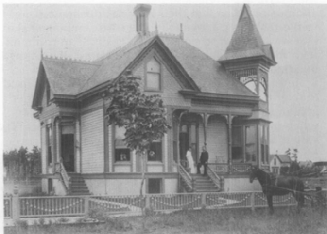
3. Readily available and inexpensive sawn shingles were used not only for roofs, but also for gables and wall surfaces. The circa 1891 Chambers House, Eugene, Oregon used straight sawn butts for the majority of the roof and hexagonal butts for the lower portion of the corner tower. Decorative shingles in the gable ends and an attractive wooden roof cresting feature were also used. Photo: Lane County Historical Society.
