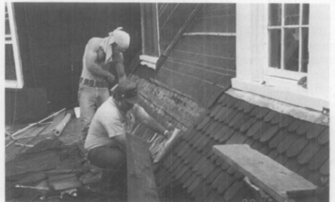
E. In order to achieve a "Class B" fire-rating, the shingles were dipped in fire-retardant chemicals and allowed to dry prior to installation. Iron oxide was added to this chemical dip to stain the shingles to match the historic red color. These coatings will need periodic reapplication.
