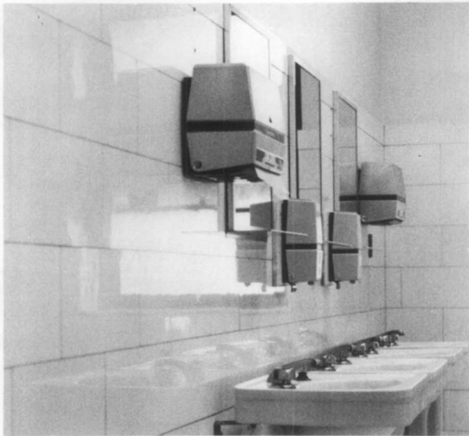
Fig. 4. White pigmented structural glass was used in this remodeling of the U.S. Custom House, Denver, Colorado. Photo: Gregory D. Kendrick.
