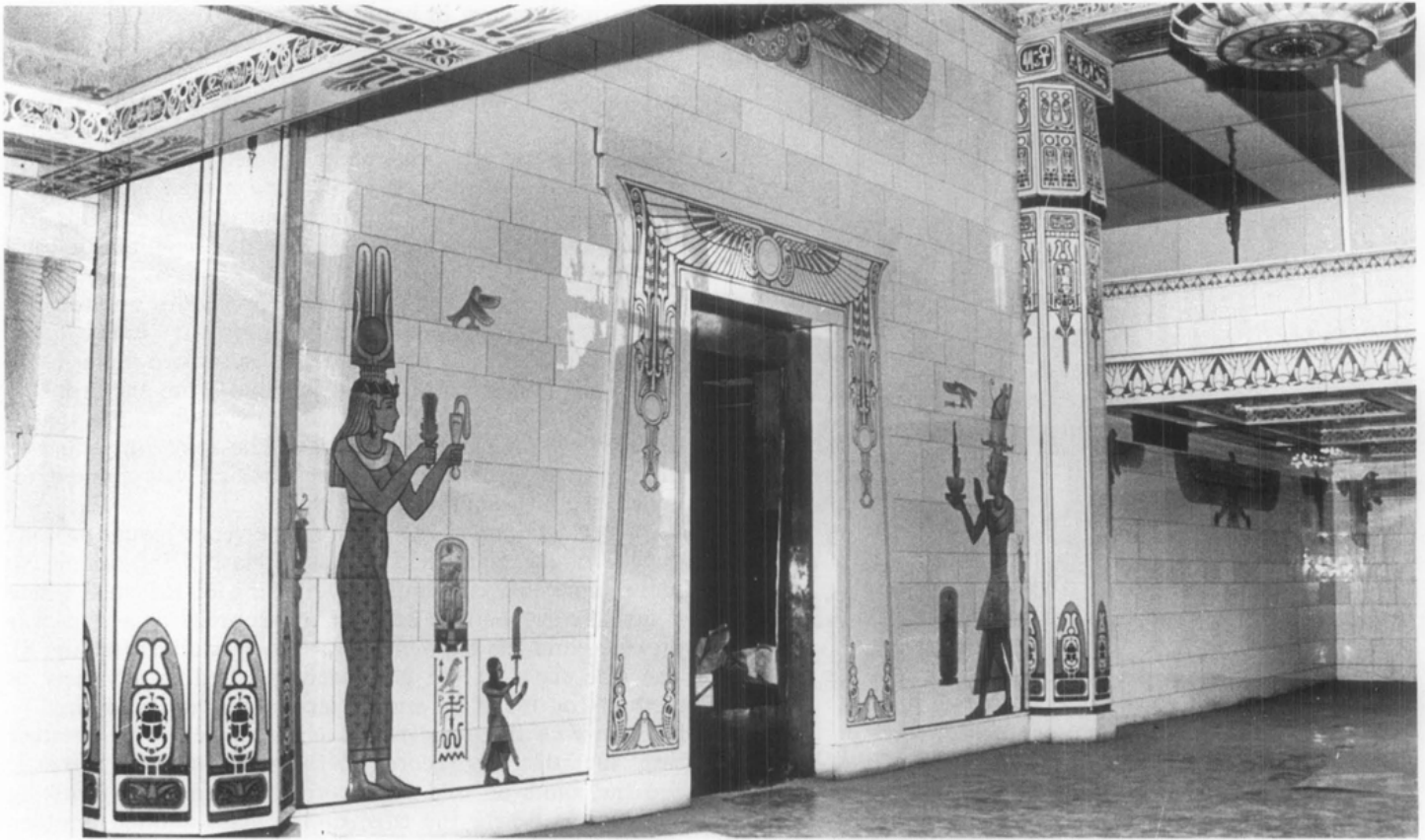
Fig. 6. Owners of the Hadley Dean Glass Company Warehouse, St. Louis, Missouri, preserved the unusual polychrome pigmented structural glass interior lobby. Photo: Paul Marshall.
