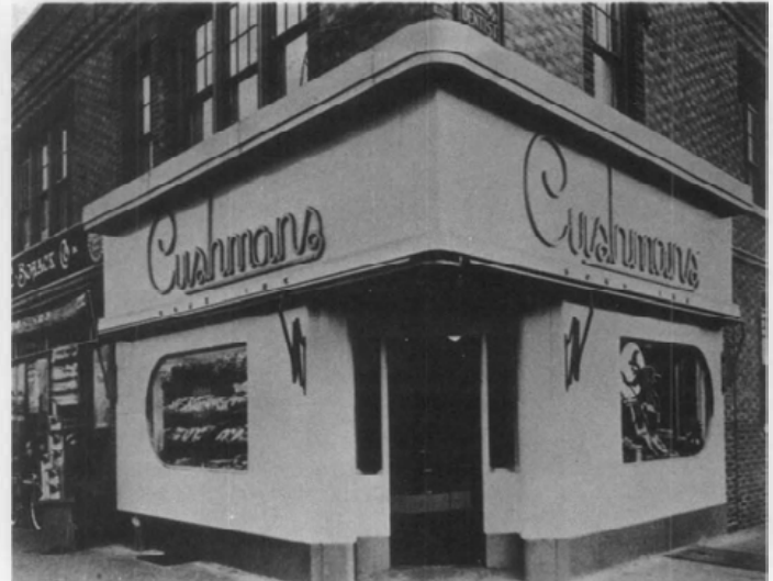
Figure 4. This storefront in New York City designed by Raymond Loewy typifies the streamlined look of the 1930's. Added to an earlier building, the front utilizes glass, stainless steel and neon to make a modern statement. This is a good example of a later storefront which has acquired significance and should be retained in any rehabilitation.
