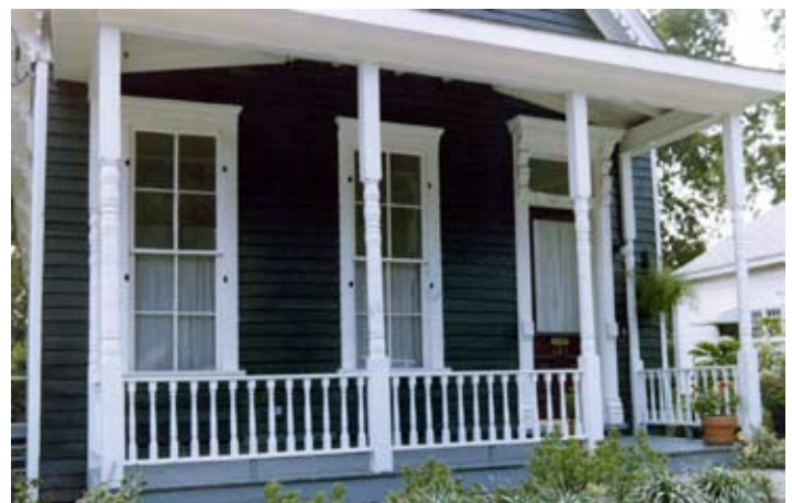
Below: To bring the project into conformance with the Standards, the original windows were reinstalled.
