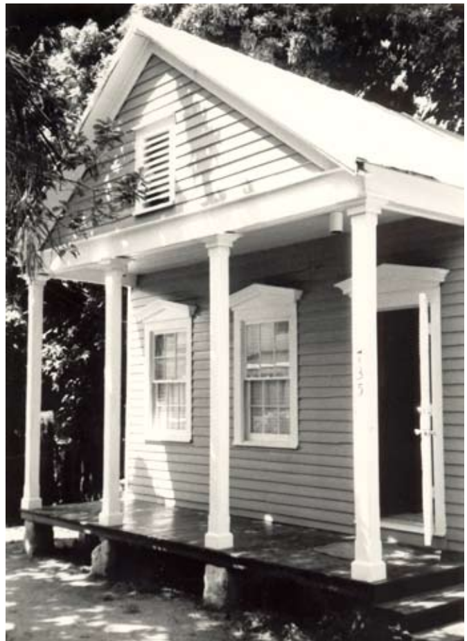
Right: The dramatic shift in appearance from a vernacular structure to a higher style building is achieved with Greek Revival posts and triangular window pediments. The building was not originally fitted with these details.
