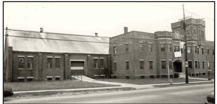
Above: The street elevation of the armory shows the head house on the right with a portion of the drill shed visible to the left.
