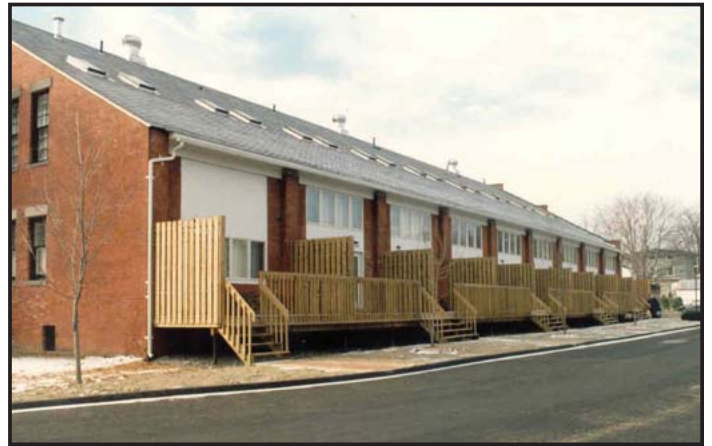
Above: The enlarged openings were infilled with wood panels, stock windows and doors (left). As a result, (right) the rear elevation of the drill house row has the residential appearance of townhouses.
