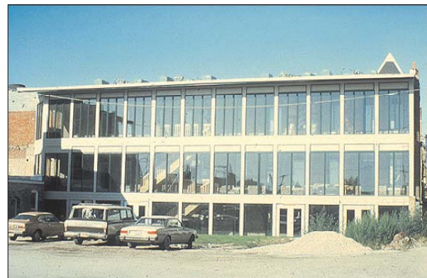
Above: The rear walls of the row houses were covered with a single glass curtain wall that is incompatible with the character of the historic houses as well as the character of the historic district.
