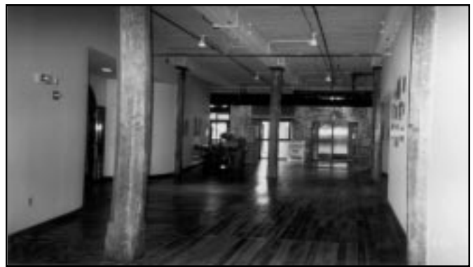
Interior after rehabilitation retains the exposed structure and finishes characteristic of the mill building with subdivision of the space for the new use.
