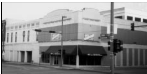
Before rehabilitation (left), the storefronts and the second floor windows were covered by plywood and metal panels. Removal of the panels revealed that the historic storefronts and windows were still intact and could be preserved (right).
