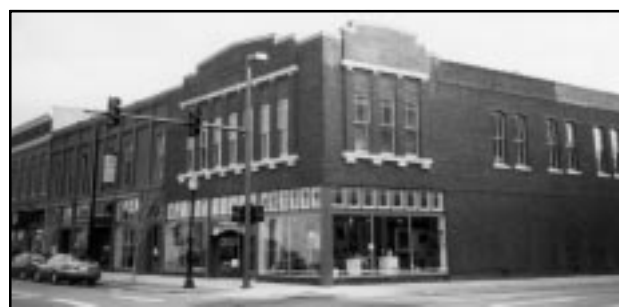
Before rehabilitation (left), the storefronts and the second floor windows were covered by plywood and metal panels. Removal of the panels revealed that the historic storefronts and windows were still intact and could be preserved (right).
