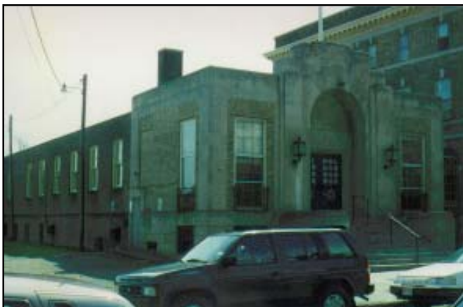
Prior to rehabilitation. Note the symmetrical head house (1938) and later rear brick shed addition (1955).
