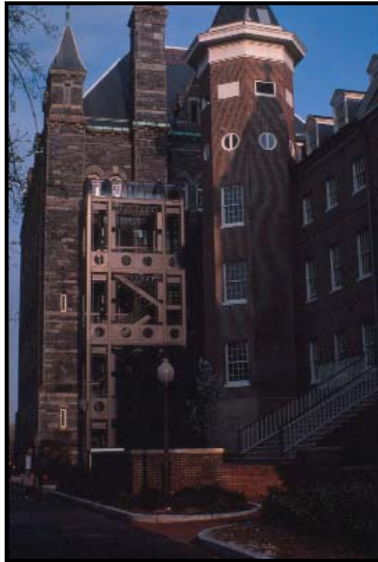
This modern, metal stair tower addition located between an existing projecting tower and articulated corner is compatible with the character of the historic structure. It is also located on the rear elevation of the building, and is not visible from major public vantage points.
