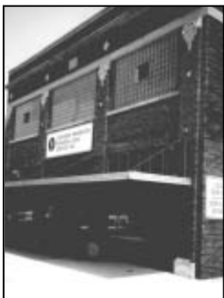
Rehabilitated dairy building.
