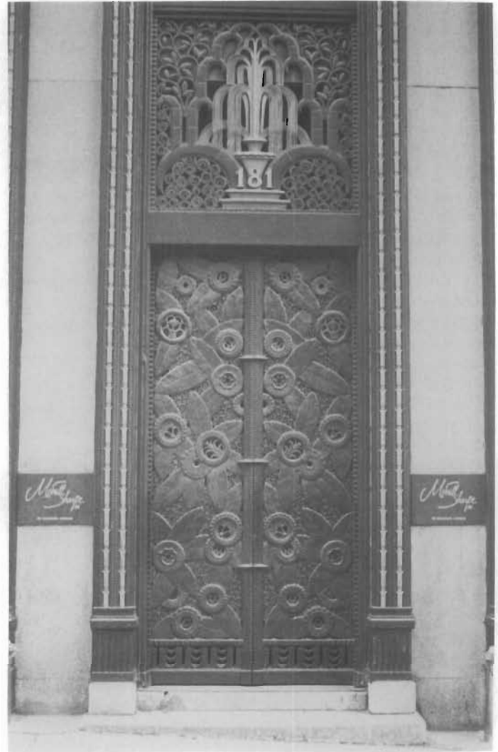
Figure 98. Cheney Brothers Silk Store (now Merrill Sharpe, Inc.), 181 Madison Avenue, New York City, 1925; Howard Greenley, designer; Ferrobrant, foundry. Originally fabricated under the direction of Jules Bouy for Cheney Brothers Silk Store. These doors were later moved in 1928 to their present location, the Madison Belmont Building. Edgar Brant of Ferrobrant fabricated the additional metalwork for the new building. Note that the parts of the frame and transom painted gold (the lighter color in the photo) are actually cast bronze, recently restored and polished. (David W. Look)
