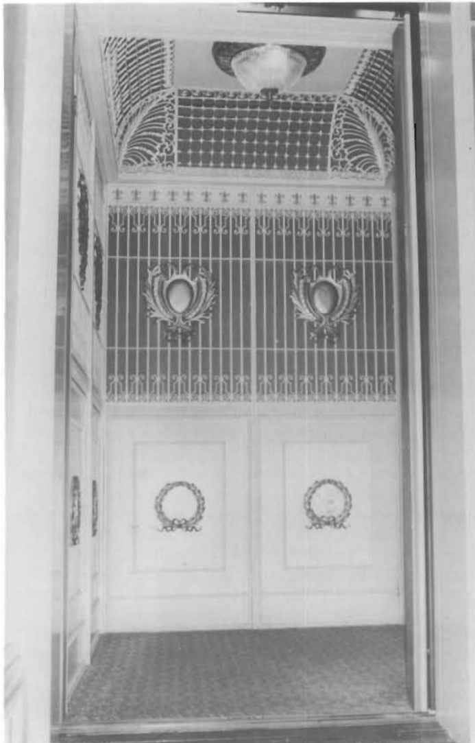
Figure 83. Cast-iron Elevator Cab, Otis Elevator Company, 1905; Pioneer Courthouse (U.S. Courthouse and Customhouse), 520 Southwest Morrison Street, Portland, Oregon, 1869-1873. To meet fire code requirements, restoration architects McMath and Hawkins installed a new fire wall inside the elevator shaft in 1973. To give the illusion of openness, the elevator grille and cab were painted a cream color, with gilt shields and wreaths; the fire wall was painted a dark gray, creating the effect of a silhouette. (Mike Henley)
