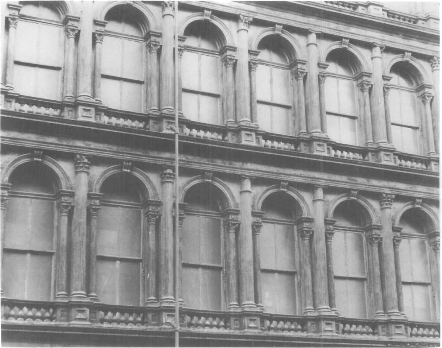
Figure 65. Cast-iron Haughwout Building, 490 Broadway, New York City, 1856; John P. Gaynor, architect; Daniel D. Badger's Architectural Iron Works of New York City. Some of the best iron front buildings stand in the SoHo area of the city. There are excellent examples of the quality and character of mass-produced 19th-century ironwork. Once foundry patterns were prepared, any number of like building fronts could be cast. The facade of the Haughwout Building consists of a single module, Palladian in character, repeated again and again. The result was an impressive design at a moderate cost. (Clover Vail)
