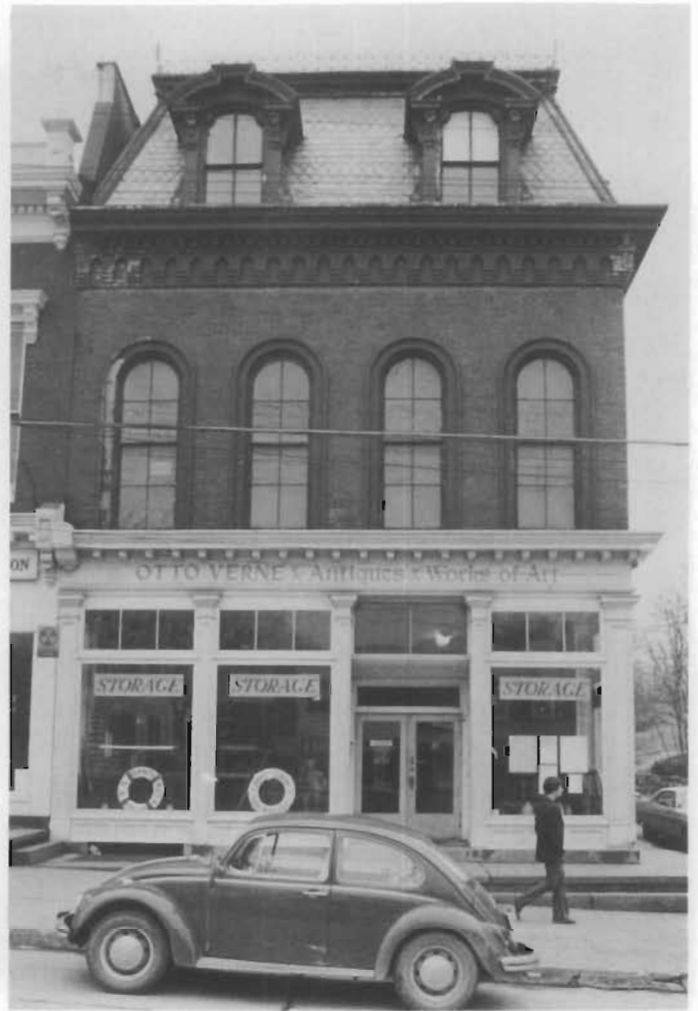
Figure 67. One-story Cast-iron Storefront, 75 Main Street, Cold Spring, New York. This modest facade is typical of cast-iron storefronts popular for decades after their introduction about 1825. Fabricated by both small local foundries and large nationally known companies, storefronts were available in a variety of styles and sizes, and could be ordered from catalogs. The slender piers and columns could support the weight of several stories, usually masonry, while providing the framework for broad expanses of glass. The open front was perfect for the display of merchandise. (Otto Verne)
