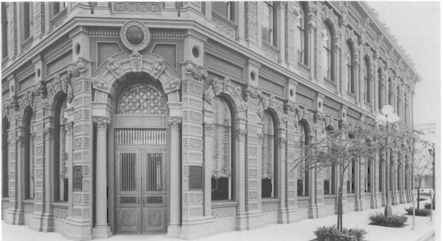
Figure 70. Ladd & Bush Bank (Branch of the U.S. National Bank of Oregon), 302 State Street, Salem, Oregon, 1869, Willamette Iron Works; addition by Skidmore, Owings and Merrill, 1967. The elaborate iron elements of this bank in Salem were a near twin to the Ladd and Tilton Bank in Portland, also cast by the Willamette Iron Works in 1868. When the latter was demolished, its iron facade was saved and later used for expansion of the Salem bank. Additional parts were cast as needed by the original foundry. Note the bronze doors which were added in 1912. (Donald Sipe)
