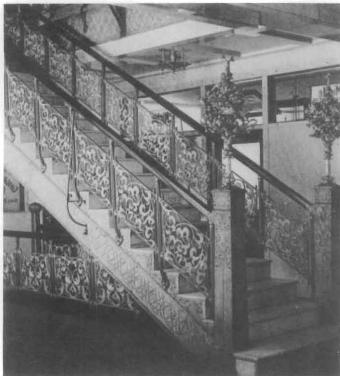
Figure 112. Cast Aluminum Staircase, Monadnock Building, 53 West Jackson Boulevard, Chicago, Illinois; Burham and Root, architects; Winslow, Brothers, Co., foundry. Although the Monadnock Building is widely known as the last skyscraper with load bearing walls, few people know that it contains the second known architectural use of cast aluminum in America. The first story staircase, including the newell posts, electroliers, balustrade railing, facias, and stringers, are all cast of aluminum. The lamps have been removed. Aluminum ventilation grilles near the exterior doors are also illustrated, but have also been removed. (plate 4, Collection of Photographs of Ornamental Iron Executed by Winslow Bros., 1893, Library of Congress)
