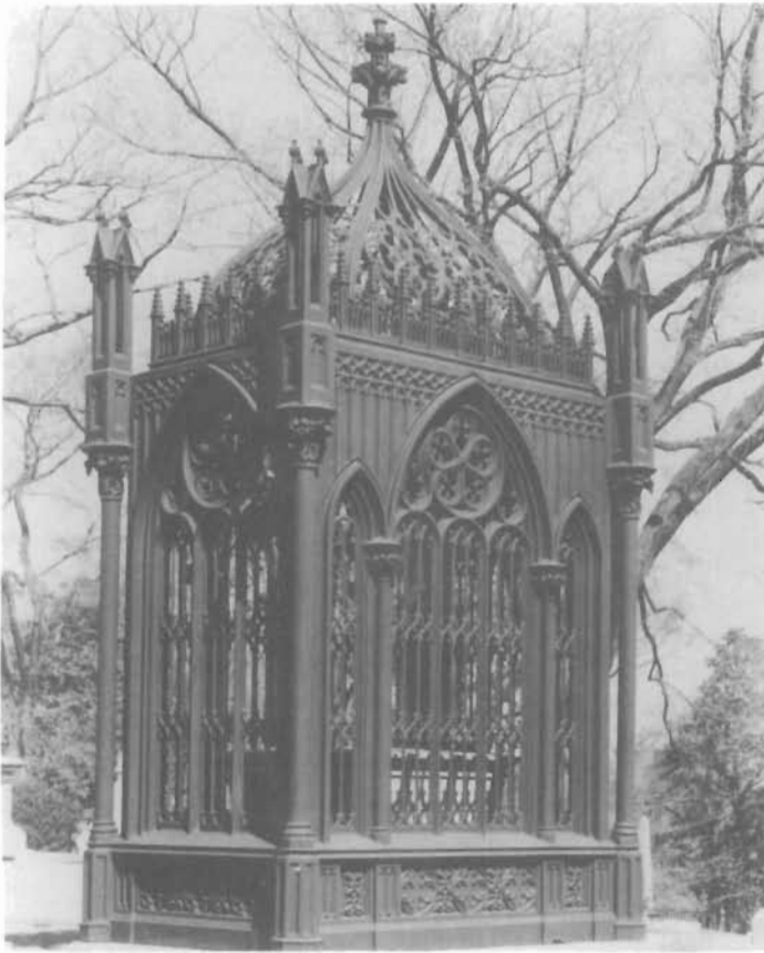
Figure 97. Cast-iron Tomb Enclosure, Grave of President James Monroe, Hollywood Cemetery, Richmond, Virginia, 1859; Albert Lybrock, architect; Wood and Perot, foundry, Philadelphia. The ceremonial enclosure of the tomb of James Monroe is a particularly fine example of cast-iron design and craftsmanship. In the 1850s the state of Virginia took steps to move Monroe's resting place from New York to his native state. The Gothic Revival design chosen for the tomb was that of German-born Richmond architect Albert Lybrock. Perhaps more important was the selection of Wood and Perot, manufacturers of ornamental iron, to prepare the patterns, make the molds, and cast the separate parts that would compose this work of art. The words "Robert Wood, Maker" can be found at the edge of the enclosure. In later years, Wood and Perot presented sketches of the tomb cover in its sales catalog. It measures 7 feet wide by 10 feet long, with a perforated canopy rising 20 feet to a finial of crockets. Four miniature corner towers enclose side panels filled with Gothic arches and trefoil patterns. (F. Heite, Library of Congress)
