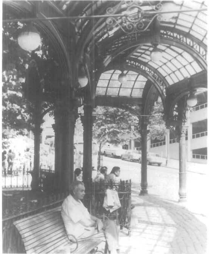
Figure 60. Iron and Glass Pergola, Trolley Station, Pioneer Square, Seattle, Washington, 1909. This station, which has become a symbol of the revival of the city's old commercial area, consists of glass panes held between ribs of wrought iron supported by cast-iron arches and columns, both of which are in compression. The wrought-iron tie rods (top of photo) take the outward thrust of the arches; thus, the rods are in tension. Iron members in tension had to be made of wrought iron because cast iron is suitable only for compressive loads. However, iron members in compression could be of either cast iron or wrought iron, whichever was more economical and convenient for the iron shop to fabricate. By the late 1960s, most of the glass in the pergola was broken and the iron was rusting. Preservationists, planners, and city officials worked together to rehabilitate Pioneer Square with the pergola as its centerpiece. Wooden patterns were carved from which sand molds were made to recast the lost and broken iron parts. With new lamps and fresh paint, the pergola was rededicated in 1973. (John Jochman, Seattle Office of Historic Preservation)
