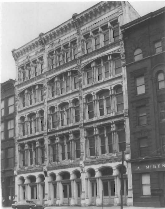
Figure 69. Iron Front Hildebrand Building, 730 Main West Street, Louisville, Kentucky, 1884; Charles D. Meyer, architect. The elaborate iron front of this five-story commercial building in the old downtown section exemplifies the advantages of cast-iron construction. The tall iron columns and colonettes between windows, slender as they are, take the weight of the materials, allowing large openings and light rooms. Iron manufacturers linked the technical requirements of their material with aesthetically appealing design, a fact which is evident even in this unrestored building. (John Albers and Preservation Alliance)
