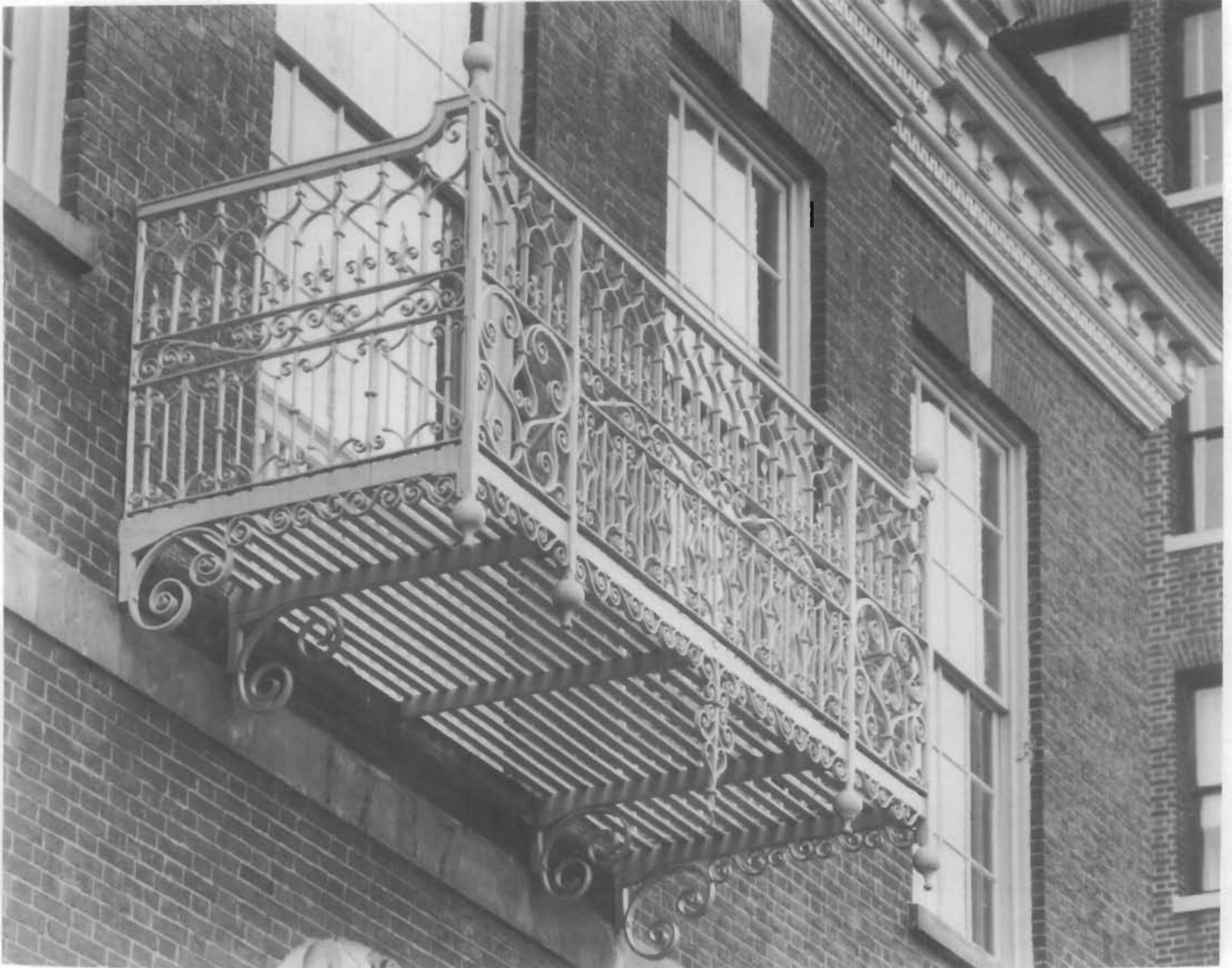
Figure 51. Wrought-iron Balcony, Samuel Wheeler, blacksmith; Congress Hall, 1787-1789, Chestnut Street at 6th Street, Independence National Historical Park, Philadelphia, Pennsylvania. Built as the Philadelphia County Court House, this building was used by the Federal Congress from 1790 to 1800. In 1961, the National Park Service removed many layers of paint from the balcony over the front door prior to its restoration. During the process, the name and date "S. Wheeler 1788" was discovered. The inscription was located on the inside of the balcony facing the window. Just a few layers of new paint have already obscured the marking. (Jack E. Boucher, NAER)
