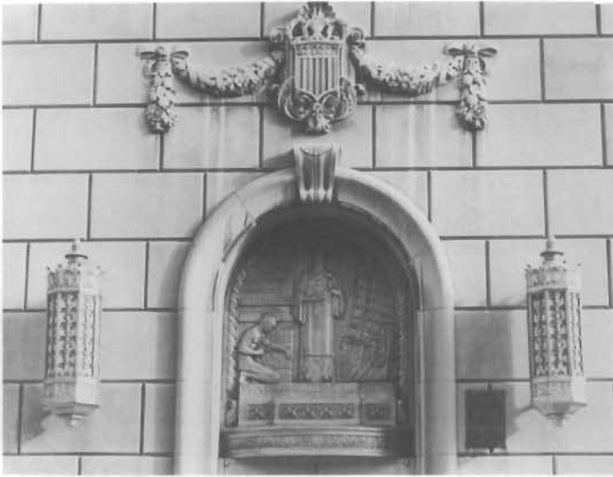
Figure 114. Aluminum Bas-Relief Sculpture in Tympanum and Lamps, U.S. Customhouse, bounded by Chestnut, Second, and Third streets, Philadelphia, Pennsylvania, 1933; Ritter and Shay, architects; Edward Ardolino, sculptor. In the 1920s and 1930s, architects frequently chose one of the white or silvery metals for their buildings; those designing in the Art Moderne, now called Art Deco style, especially considered gold or bronze colored metals "old-fashioned." The highly stylized bas-relief mural in the tympanum is flanked by cast aluminum and glass lamps. (Esther Mipaa)
