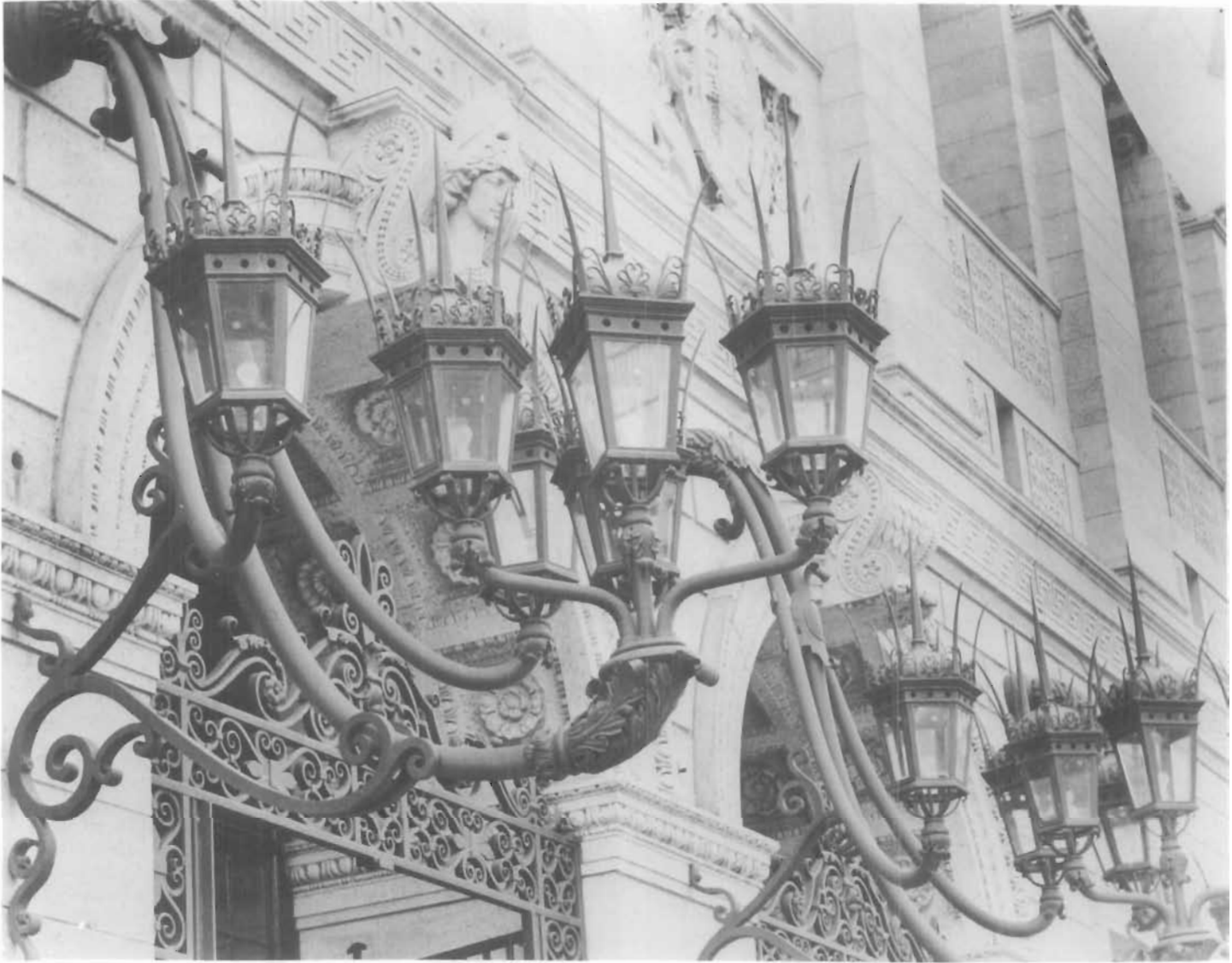
Figure 93. Iron Lamps, Boston Public Library, Copley Square, Boston, Massachusetts, 1895; Charles Follen McKim, architect. The Boston Public Library contains many forms of metal ornamentation: bronze doors by Daniel Chester French, wrought-iron gates and grilles, and Strozzi-type wrought- and cast-iron lamps which flank the three entryways. Repeated casting from the same molds made ornamentation worthy of a Renaissance palace affordable in the 19th century. (Esther Mipaas)
