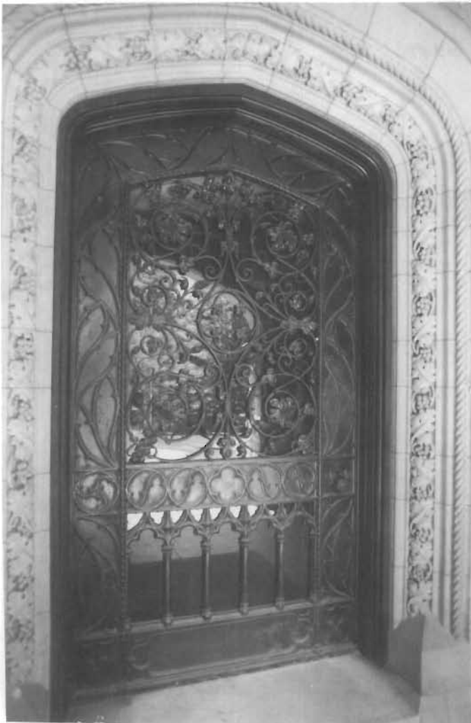
Figure 57. Wrought-iron Door, Joslyn Castle, 3902 Davenport Street, Omaha, Nebraska, 1902-1904; Winslow Bros., foundry, Omaha. The one-ton iron door to the entrance hall of this Scottish baronial-style mansion is precision balanced and swings easily. A hand-forged wrought-iron grille consisting of scroll and vine motifs is set in Gothic cast-iron framing. (Robert Peters)
