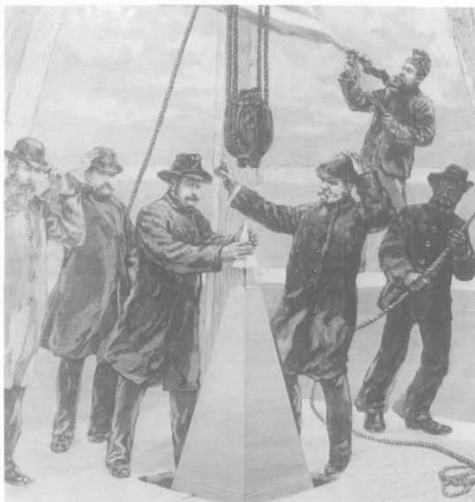
Figure 111. The Setting of the Aluminum Tip on the Washington Monument, Washington, D.C. The first architectural use of aluminum was the small pyramidal cap of the Washington Monument, which was set in place on December 6, 1884. At that time, aluminum was still considered a precious metal. (Engraving in Harper's Weekly, December 20, 1884; Martin Luther King Library)
