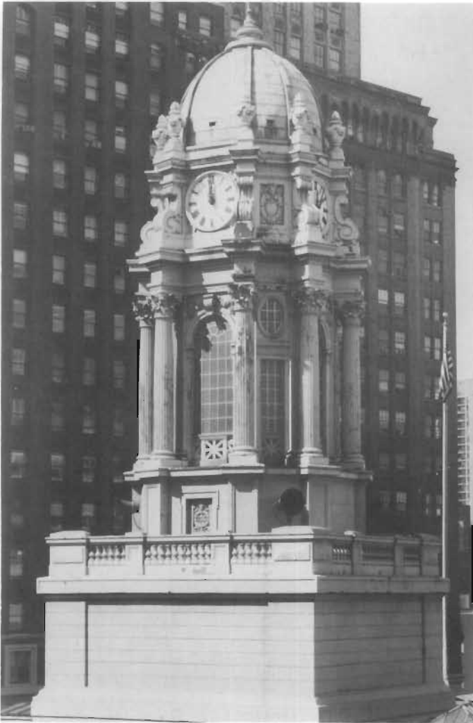
Figure 76. Cast-iron and Sheet-iron Cupola, Designed by C. W. and A. A. Houghton, architects, 1898; Hecla Ironworks; Borough Hall, 209 Joralemon Street, Brooklyn, New York, 1846-1851; Gamaliel King, architect. After the Old Brooklyn City Hall burned in 1895, it was rebuilt within the masonry shell, and a cast-iron and sheet-iron cupola replaced the wooden one that had been destroyed in the fire. It is typical of many such cupolas throughout America. (Esther Mipaas)
