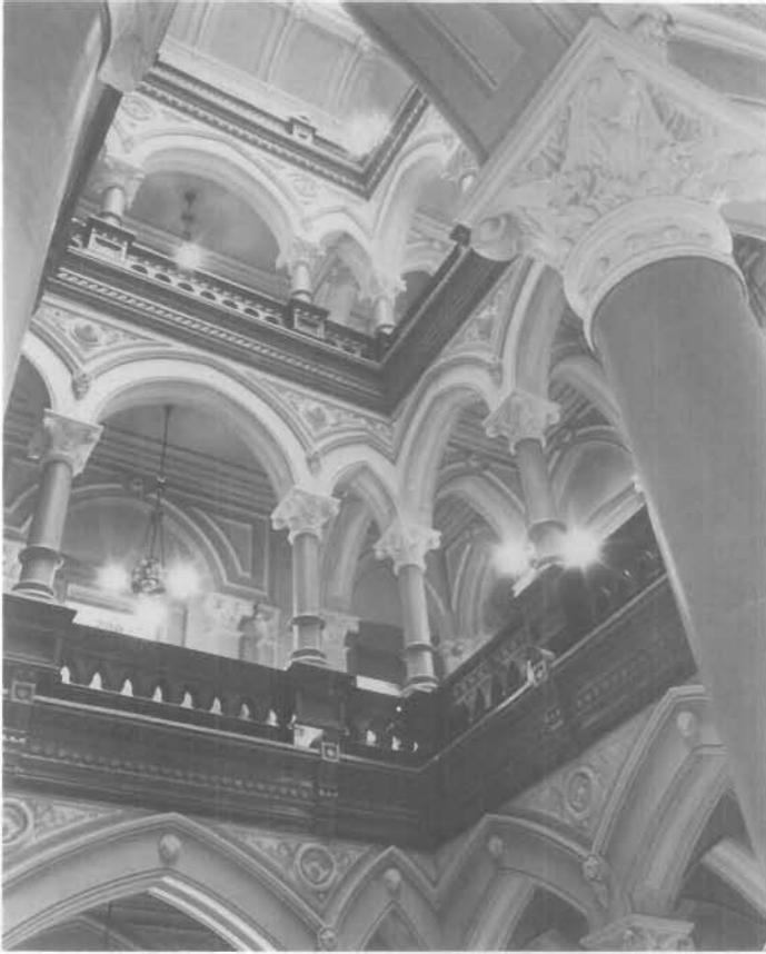
Figure 78. Cast-iron Light Court, Old City Hall, bounded by 10th, Broad, 11th, and Capitol Streets, Richmond, Virginia, 1886-1894; Elijah E. Myers, architect. The great central light court with its tiers of enriched cast-iron columns, spandrels, railings, and brass fixtures ranks as one of the most impressive municipal interiors in America. In imitation of stone, the cast iron has a massive, solid quality consistent with the character of the exterior masonry. (William Edwin Booth)
