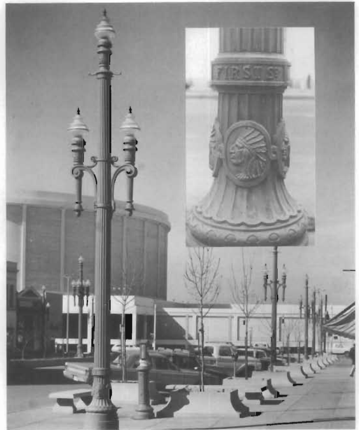
Figure 92. Cast-iron "Indian Head" Lamps, Salt Palace Complex, Salt Lake City, Utah. (a) Electric street fixtures began to replace gas fixtures in the 1880s; many of the ornate electric street lamps were erected about the time of World War I. (b) Salt Lake City put up cast-iron street lamps with Indian head medallions on the bases. With the recent revival of interest in the downtown area, the Utah Power and Light Company refurbished the surviving lamps and had others made. (Hal Rumel Studio; Utah Power and Light Co.)
