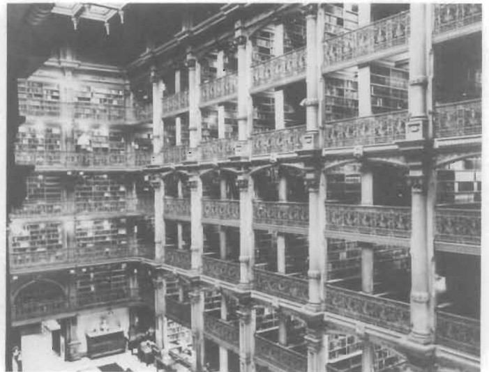
Figure 77. Cast-iron Interior, Peabody Institute Library, Mount Vernon Place, Baltimore, Maryland, 1857-1878; Edmund George Lind, architect; Bartlett, Robbins and Co., Architectural Iron Works, Baltimore. A gift from the philanthropist, George Peabody, who started his career in Baltimore, the Peabody Institute included a library which is virtually all cast iron and glass. Although the building's exterior is a traditional Renaissance design in stone, the most innovative materials of the time were used on the interior to safeguard the collection of books and manuscripts from fire. The central area of the library is surrounded by five floors of cast-iron galleries and is covered by one great skylight of glass set in an iron frame. The floors of the five decks are of iron inset with blocks of translucent glass. The decks are supported by cast-iron piers with applied two-story fluted pilasters rising in three tiers from floor to roof. (Peabody Library)
