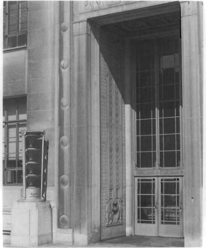
Figure 115. Aluminum Doors and Lamps, U.S. Department of Justice, Ninth and Constitution Avenue, NW, Washington, D.C., 1934; Zantzinger, Boris, Medary, architects; Carl Paul Jennewein, sculptor. The monumental doors, fabricated of cast lions and rolled sections of aluminum riveted together, are opened back into pockets of the walls of the entrance showing the inner set of aluminum and glass doors and transom. Flanking the entrance are cast aluminum lamps with stylized eagles, buffaloes, and dolphins. The work was executed by Anthony D. Lorenzo. (David W. Look)
