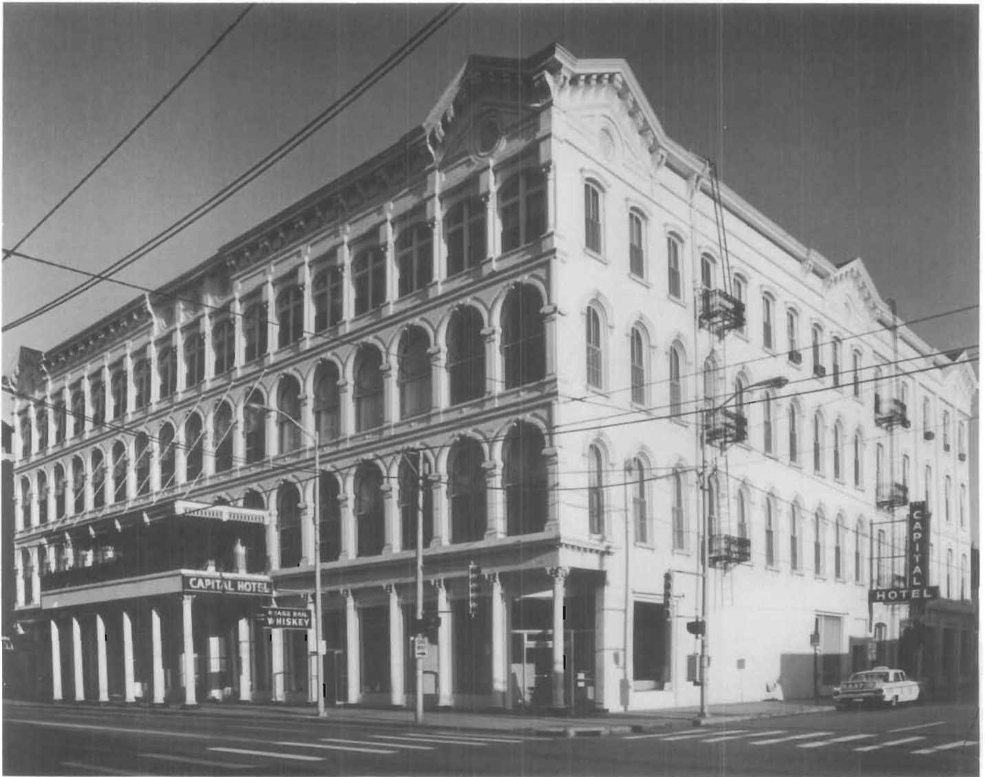
Figure 68. Cast-iron Facade, Capital Hotel (originally the Denkla Office Building), 117 West Markham Street, Little Rock, Arkansas, 1873. The Italianate office building was converted in 1877 into a hotel. Being located near the state capitol, it became popular with politicians and was often used as campaign headquarters. Note the difference in window size in the facade and the masonry sidewall. The larger windows of the cast-iron front provided a great deal of natural light, which the building's original use (offices) required. Although not apparent from a distance, the top story of the front facade and the cornice are pressed sheet metal, probably galvanized iron. (Earl Saunders)
