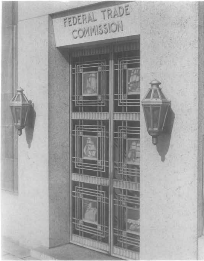
Figure 108. Stainless Steel Gates, Lamps, and Lettering, Federal Trade Commission, Sixth and Constitution Avenue, NW, Washington, D.C., 1937; Bennett, Parsons, Frost, architects; William McVey, sculptor. During the 1930s stainless steel was frequently used for monumental doors and ornamental gates on government buildings. Noted sculptors were employed to design custom ornamental metalwork. The lamps, lettering, and window grilles (not shown) are all stainless steel. (David W. Look)
