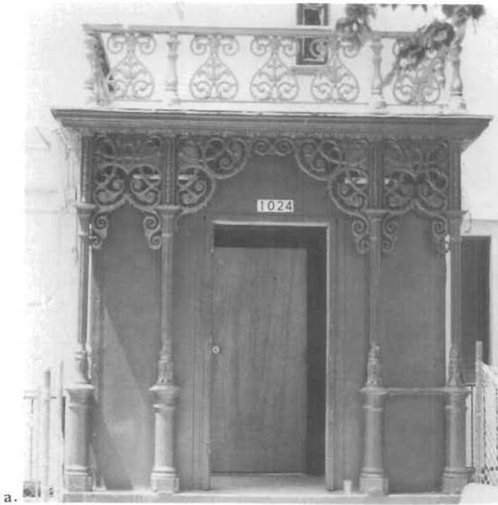
Figure 88. Cast-iron Veranda, Zephaniah Jones House, 1024 10th Street, NW, Washington, D.C.; Janes, Kirtland and Co., foundry. (a) It is a rewarding experience to see an advertisement for an architectural feature in a foundry catalog, then to discover the original model is still extant. (b) This veranda appears in Janes, Kirtland and Company's 1870 catalog of ornamental ironwork. The caption reads, "Verandah made to order for Z. Jones, Esq. of Washington, D.C." The veranda, in need of repair, remains on the Jones House over 100 years after its installation. (David W. Look)
