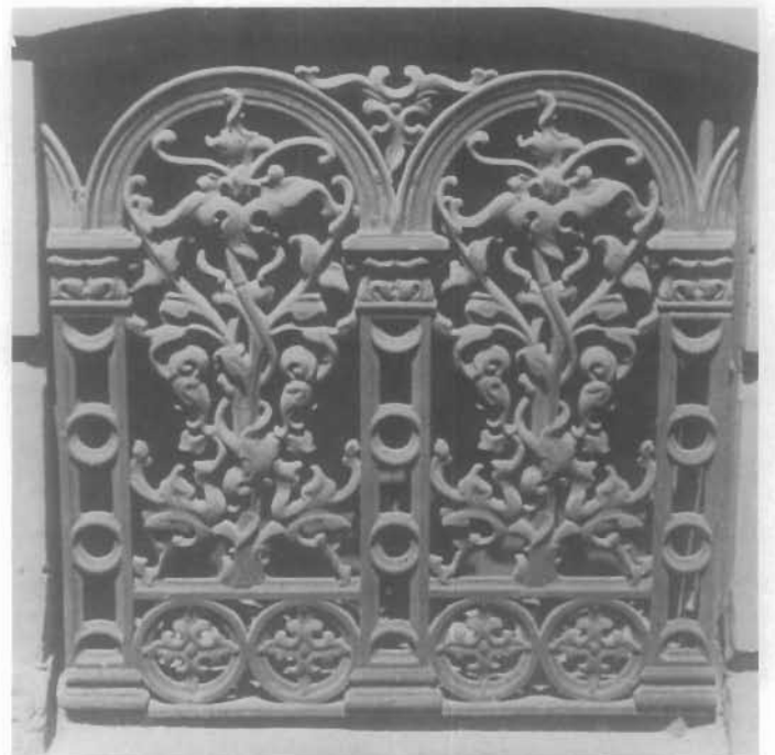
Figure 85. Cast-iron Cellar Window Grille, Matthew Quay House, northeast corner of Spruce and 11th streets, Philadelphia, Pennsylvania. Although little noticed, there is a seemingly endless variety of decorative cellar window grilles in Philadelphia. With the first-floor level several feet above grade and the sidewalks often extending right up to the facade, these articulated iron grilles were installed to protect exposed cellar windows while still allowing ventilation. The grille photographed here displays a motif of cast-iron vines set in a pair of arched panels. (Harley J. McKee, FAIA)
