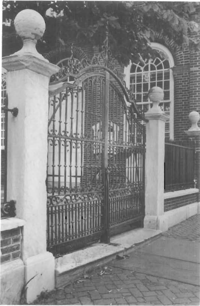
Figure 52. Wrought-iron Gates, Samuel Wheeler, blacksmith; Christ Church, 22-26 North Second Street, Philadelphia, Pennsylvania, 1727-1744; attributed to Dr. John Kearsley, builder-architect. (a) The wrought iron was heated, hammered, bent, and twisted to achieve the various parts of the design. The verticals were split and then bent to form the scrolls, rather than bent and attached to the verticals. (b) Like the balcony on Congress Hall (see figure 51), these gates are signed and dated; "S. Wheeler 1795" appears on the edge of the gate, seen only when the gates are open. (Jack E. Boucher, NAER)
