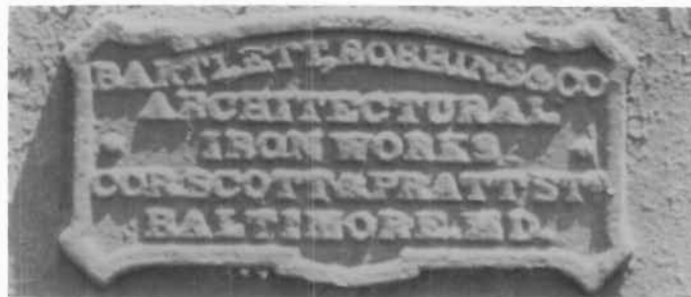
Figure 71. Foundry Label: "BARTLETT, ROBBINS & CO., ARCHITECTURAL IRON WORKS, COR. SCOTT & PRATT ST., BALTIMORE, MD." Foundries often attached labels to their work, a tradition started by bronze founders. A combination of pride and promotion, foundry labels can be found on architectural ironwork all over the country. This label appears on a building in downtown Baltimore. For some years the firm's name was Hayward, Bartlett and Co., under which it cast iron fronts for an attractive row of stores in Richmond, Virginia, recently restored as an office building. (David W. Look)
