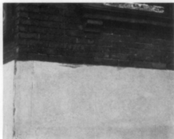
Parging over brick. Photograph: National Park Service.
