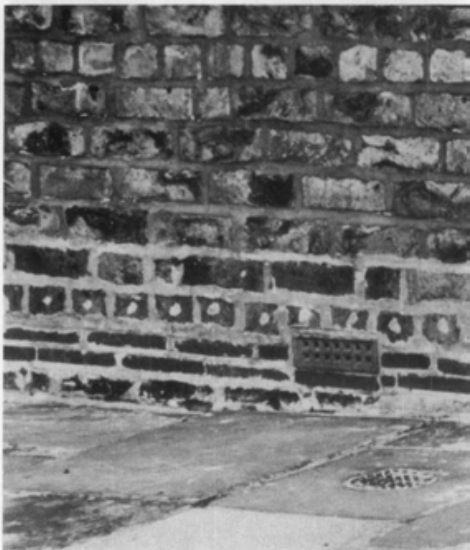
The horizontal row of white dots in the brick headers indicates that a chemical dampproof course has been injected. Photograph: Baird M. Smith, AIA.
