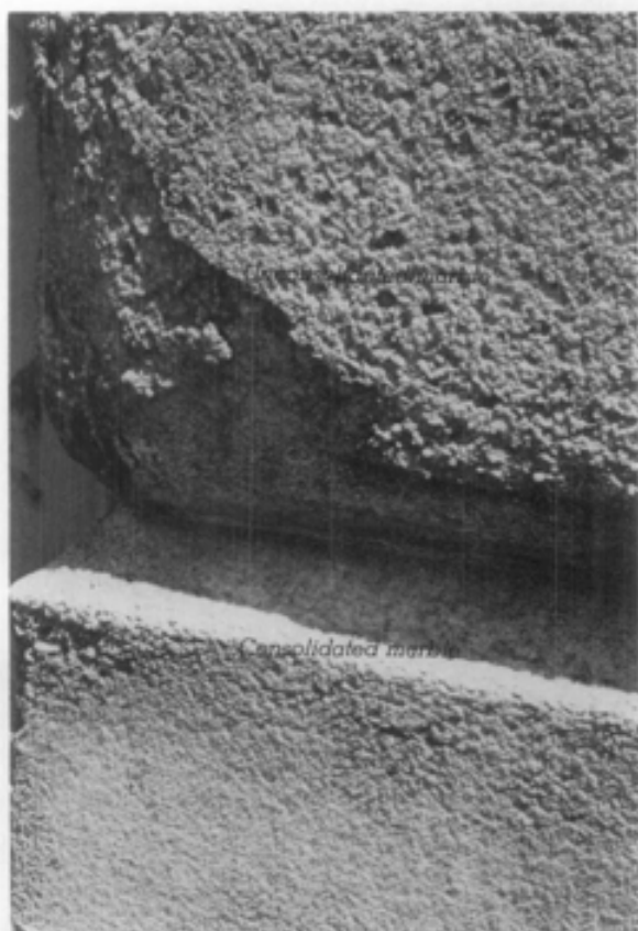
A barium hydroxide consolidant (nearly invisible in the photograph) has been applied here in an attempt to consolidate this sugaring marble. Photograph: Christina Henry.
