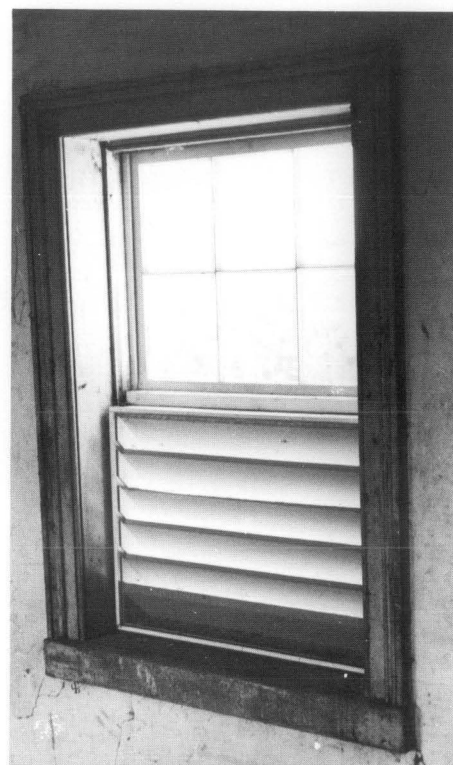
Figure 5. Screening was attached to the back side of the louvers to prevent the recurrence of insect, bird, and rodent infestation. Photo: Charles Fisher
