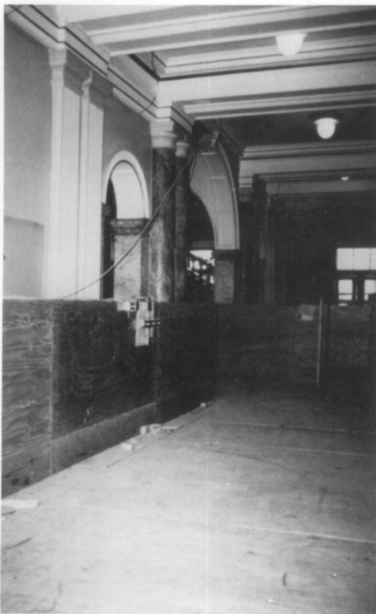
Figure 5. To provide for adequate floor protection in the New Jersey State Capitol, this area was swept clean, then covered with polyethylene sheeting to protect against spills and dirt abrasion. Fiberboard (1/2" thick) was placed over floors and the joints sealed with tape. Finally 1/2" plywood was laid with all joints taped. This floor protection system has been successful over many years of use and is recommended in major construction areas, and where tile, marble, parquet wood, or other historic flooring is involved. Photo and drawing: Ford Farewell Mills and Gatsch Architects.
