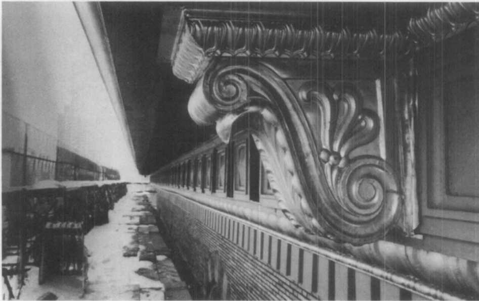
Figure 9. The new modillions, shown here in an installation test, were the same size as the originals but not precisely the same design. Had the difference in appearance been discernible from the street below, matching pieces could have been manufactured at an additional cost. Photo: Michael Devonshire.
