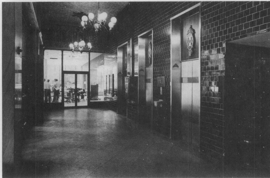
Figure 3. First floor elevator lobby, c. 1962. Modifications included reduction in number of elevators and addition of masonry enclosure around open elevators and main building stair. Photo: Cannon.
