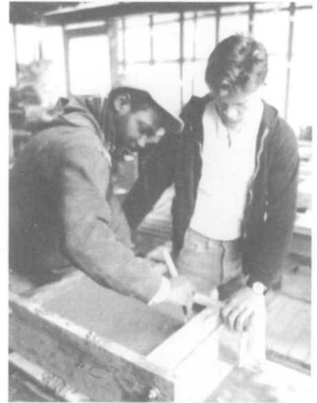
Figure 7. The workmen shown here are cutting the air bubbles from the sides of the mold using a cake spatula during the first 10 seconds of the vibration process. Photo: James Smith
