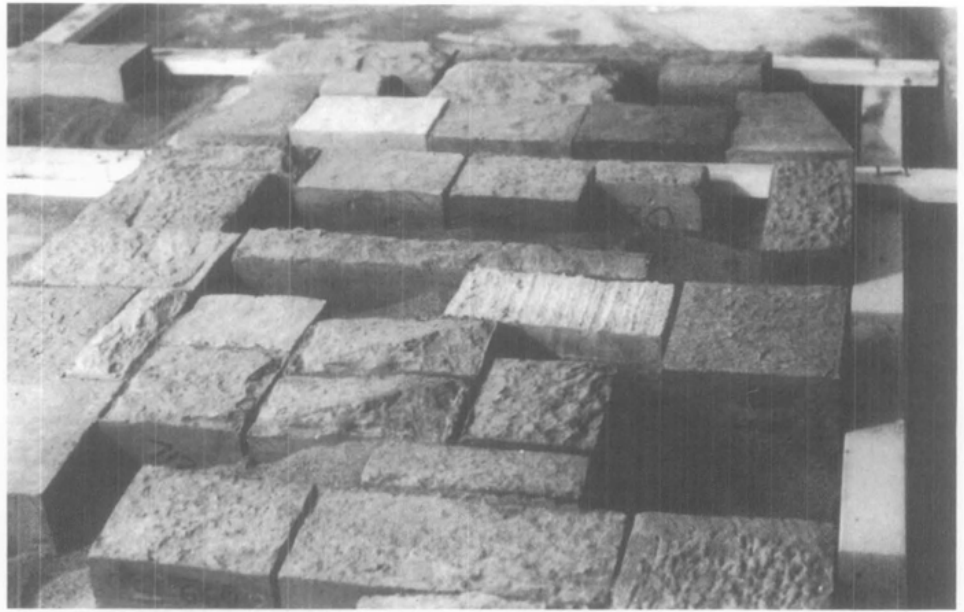
Figure 9. Using the measured drawings as a guide, the pre-cast units were assembled in the staging area on top of 4 inches of sand prior to their installation on the facade. Photo: Robert Powers
