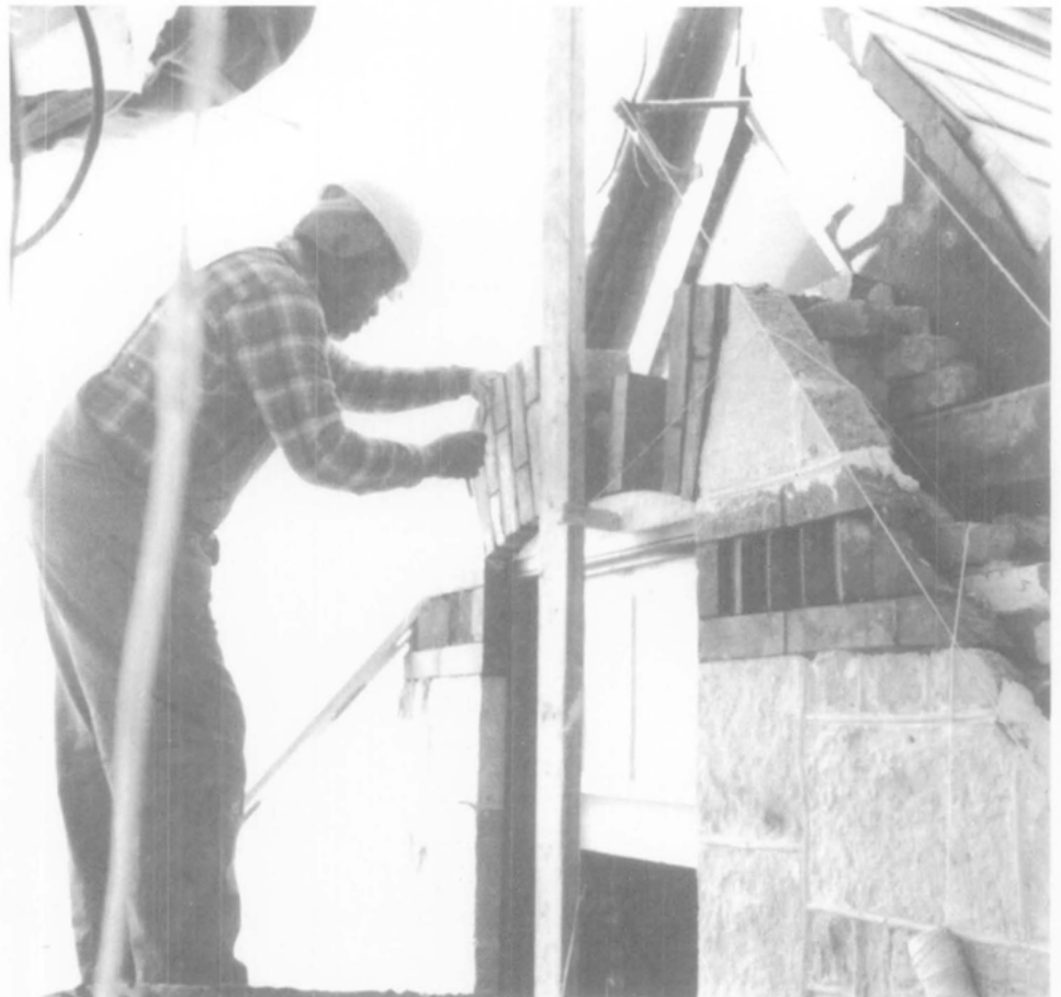
Figure 10. The new pre-cast units were hoisted up the scaffolding on wide belt slings with an electric winch, and installed in place using a portland cement-based mortar appropriate for cast-concrete. The original bricks were relaid with a more traditional lime-based, dark-colored mortar. Photo: James Smith
