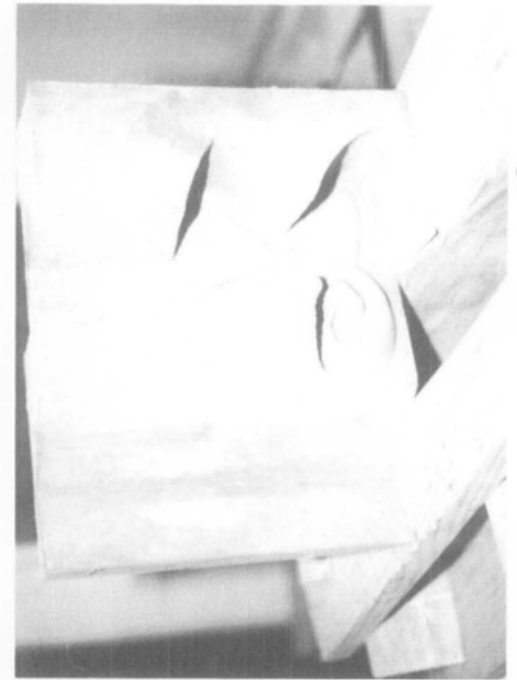
Figure 6. A rubber impression made from this latex casting mold then provided the mold into which the concrete was poured to create the new pre-cast units. Photo: James Smith
