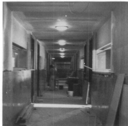
Figure 4. The window-like openings introduced by the wall removal greatly reduced the "tunnel" quality of the corridor and noticeably opened up the office spaces. Photos: Chris Henry.
