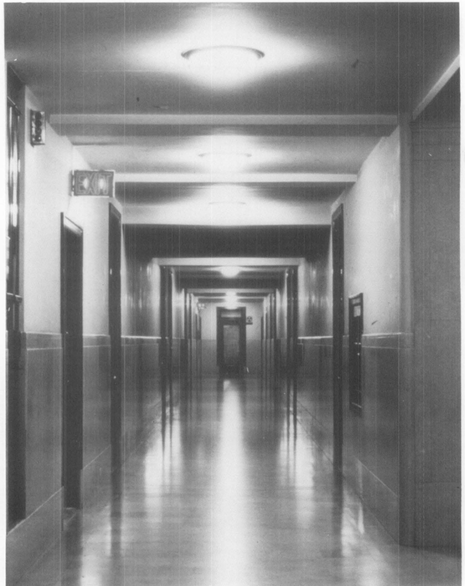
Figure 2. The central corridors, which help define the historic office plan, retain a high degree of architectural integrity, including the marble wainscoting and original light fixtures. Photo: Tom Crane.
