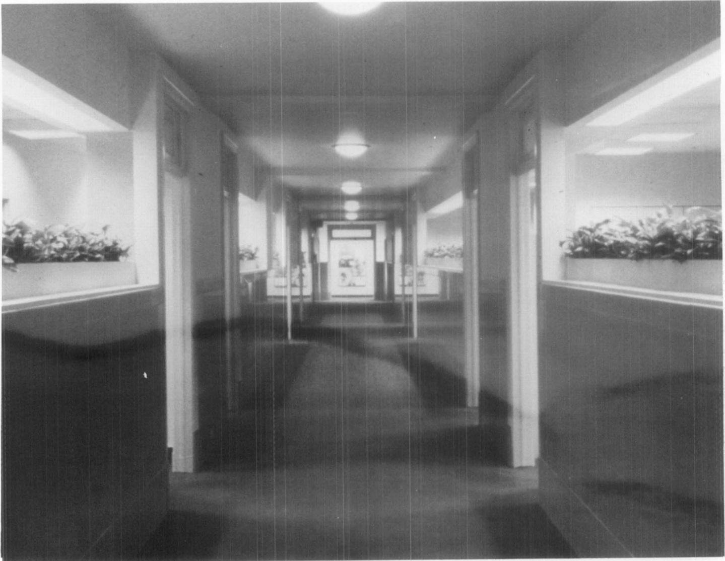
Figure 7. The historic double-loaded corridor plan, most of the hallway's significant features and sense of space have been retained while utilizing an innovative design to achieve a more open, flexible office plan. Photo: Tom Crane.
