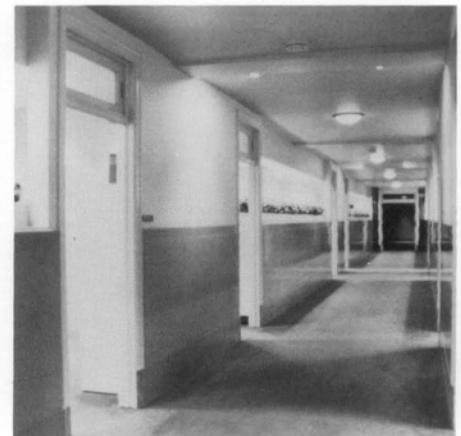
Figure 4. The window-like openings introduced by the wall removal greatly reduced the "tunnel" quality of the corridor and noticeably opened up the office spaces. Photos: Chris Henry.
