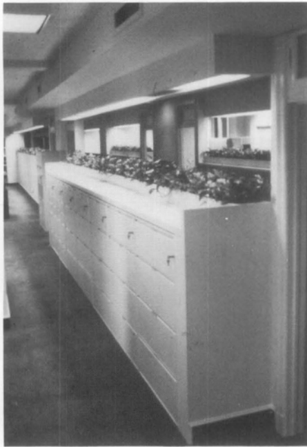
Figure 5. Banks of file cabinets and shelving were set flush against the existing wall and enclosed on the sides and tops. Photo: Nelson & Associates.
