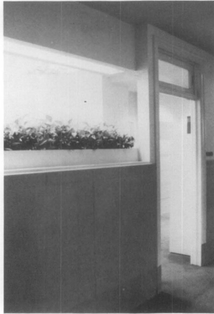
Figure 6. An alternate detail retaining the soffit at the original corridor wall plane would achieve a greater visual continuity of the historic walls, ceilings and doorways. Photo and Drawing: Chris Henry.
