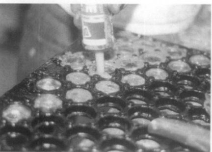
Figure 9. A caulking gun helped workers apply the waterproof epoxy grout around the lenses.
