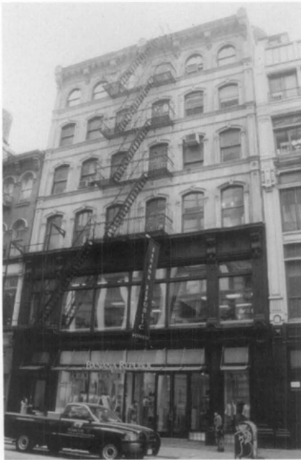
Figure 1. A cast-iron storefront was added to 552-554 Broadway in 1897. The storefront included a fifty-four foot long assembly of cast-iron vault lights set in the sidewalk. Glass lenses in the panels allowed light to enter the basement area, increasing rentable space for the building owner.
