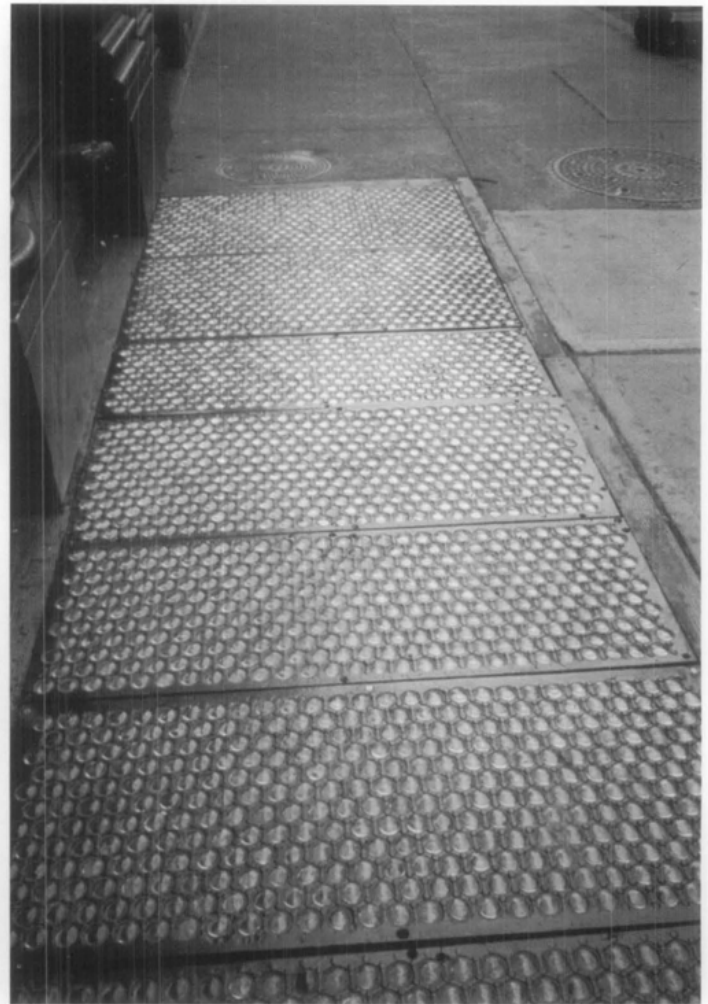
Figure 14. The restored panels after work was completed.
