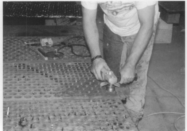
Figure 5. Workers removed any remaining corrosion, grout and other contaminants with hand chisels and power-operated wire brushes.
