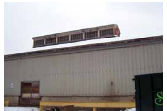
[12-14] Roof monitors provide natural light in historic industrial buildings
