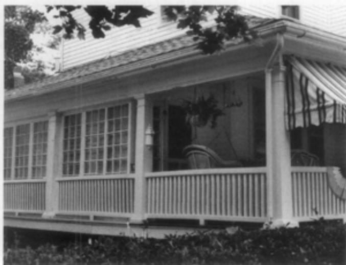
Figure 15. A traditional technique of porch enclosures still used today involves the insertion in each column bay of one or more glass enclosures set in wood frames. This enclosure is properly set back an entire porch bay from the front of the house and utilizes traditional light divisions and wood frames. The balustrade, added here for illustration purposes, shows the importance of retaining this linear feature within the enclosed bays. Photo: Charles Fisher.
