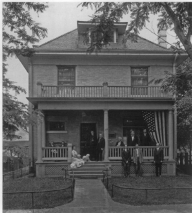
Figure 4. Celebrating the 4th of July in 1912, this gathering of family and friends reflects the popularity of the porch as a social gathering place. While not overly ornate, each detail of the porch from the roof balustrade to the turned columns to the simple lattice work facing the deck contributes to its character, creating in effect the dominant architectural feature of the building. Photo: © Utah State Historical Society
