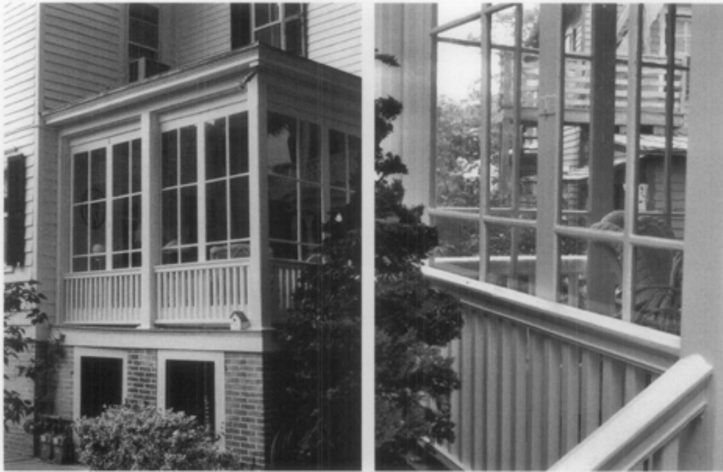
Figure 12. This old porch enclosure, located on the back side of a house, has acquired significance over time and is remarkable both in the appropriateness of its detailing for use by others today, as well as its high degree of maintenance. The enclosure is set behind the columns; the balustrade has been retained; and the light divisions and the size of the glass panes echo that of the windows above. Within each bay there are two well-crafted, inward swinging doors, providing for greater seasonal use of the porch. Photos: Charles Fisher.
