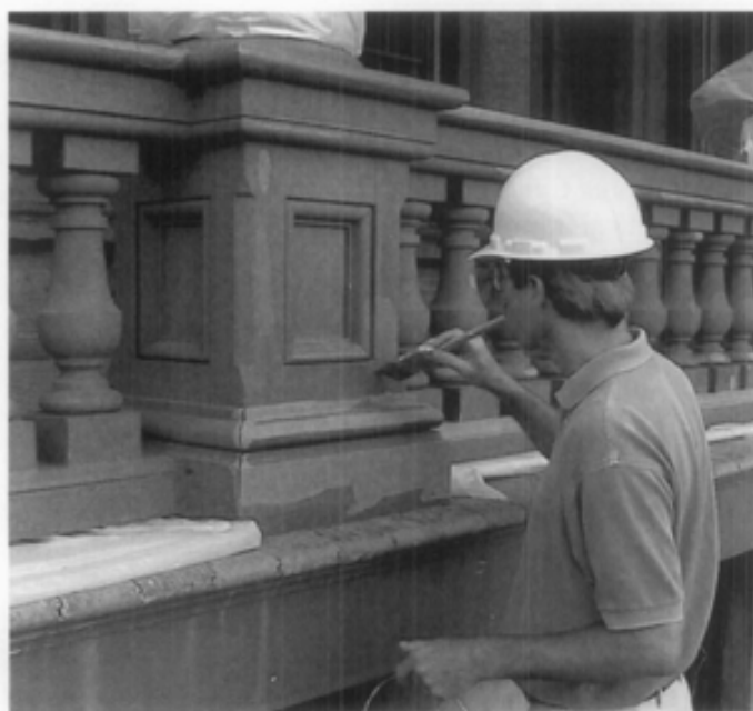
Figure 8. Decay can start when wood is left exposed to the weather or where joints open up. An inexpensive way to extend the life of the existing porch paint without jeopardizing the historic material is spot paint and caulk where needed every year or two. This cost-effective procedure is particularly effective in maintaining wood porches where the exposure to weathering is high. Photo: John Leeke.
