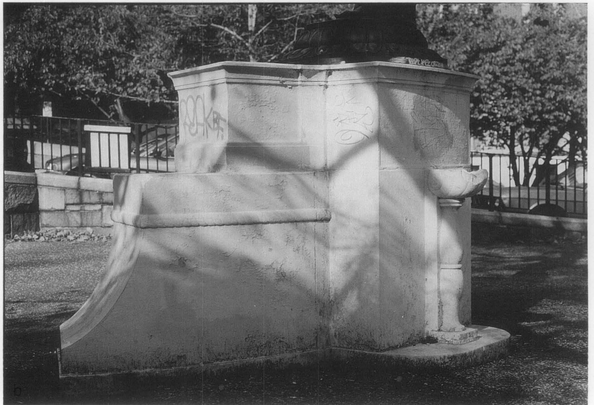
Figure 12. (a) Graffiti that was overpainted has been exposed here as a result of the coating's failure. The uneven edges where the overpainting has peeled away will make inconspicuous touch-up difficult. (b) The unsightliness of graffiti bleeding through layers of cracked and peeling paint makes an obvious point that using a pigmented coating was not an appropriate maintenance technique for this stone sculpture base. Photos: (a) Martin E. Weaver, (b) Judith M. Jacob.
