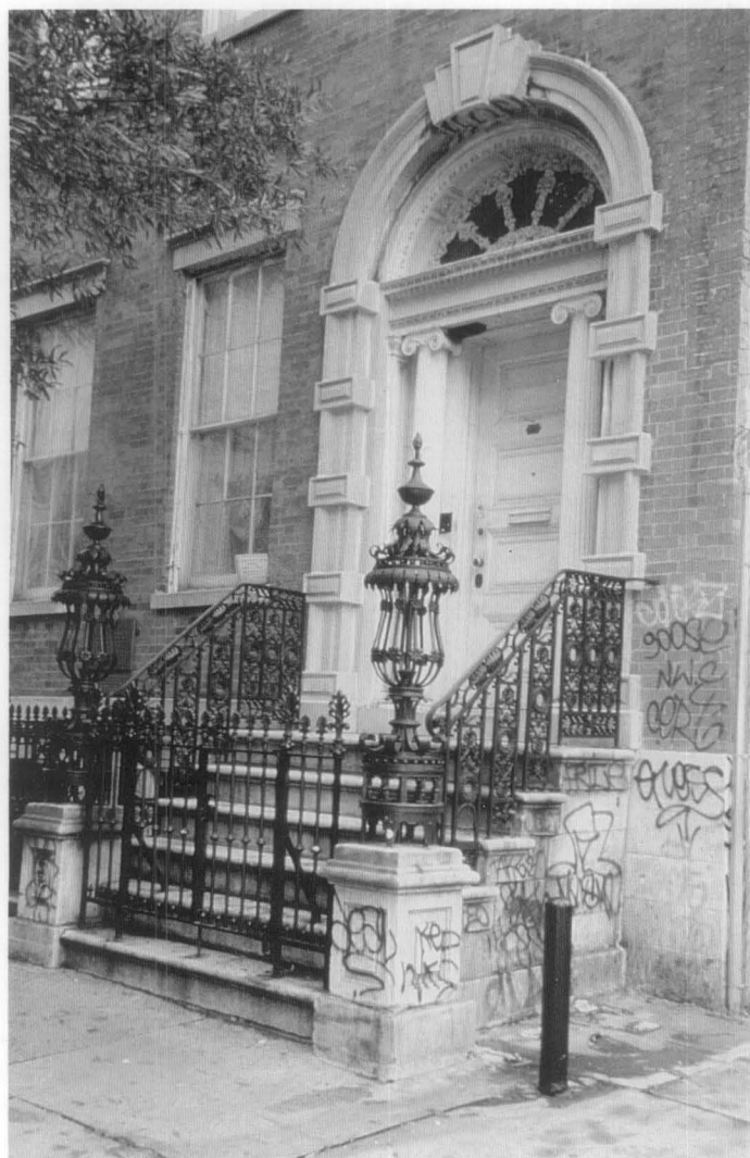
Figure 1. Many stones resemble others, and even concrete can sometimes be mistaken for stone. The stone trim on the Old Merchant's (Seabury Tredwell) House (1832), in Greenwich Village, New York City, is documented as Vermont marble. After establishing the stone type, cleaning methods should be tested in a discrete location in order to determine the most effective means of removing the graffiti without damaging the stone. More than one kind of removal technique may be required when both stone and brick require cleaning. Photo: Mark A. Weber
